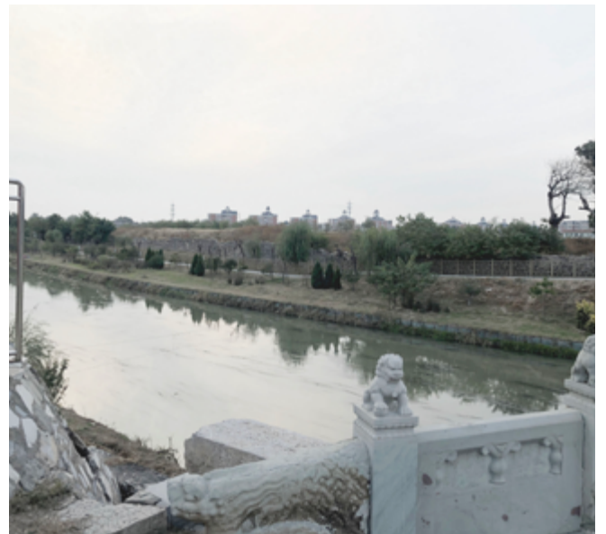
[3] The Grand Canal in Zhangjiawan, Tongzhou district Photo taken by author
