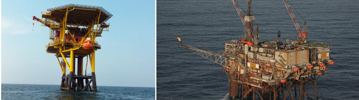
Figure 2.1: The Ameland-Westgat-1 is the smallest steel jacket of about 100 tons, and the Ninian South, 43,700 tons, is the heaviest fixed steel jacket in the North Sea (Pictures from *tekla.com* and *upstreamonline.com* respectively)
