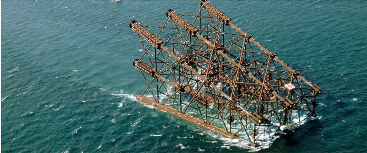
Figure 3.7: Few jackets are installed as so-called self floaters. The ballasted legs could be repaired and purged with air to refloat the jacket. Picture from *shell.co.uk*.
