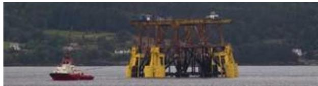
Figure 1.6: Frigg DP2 jacket towed to shore via re-float method (*picture from offshore-mag.com*).
