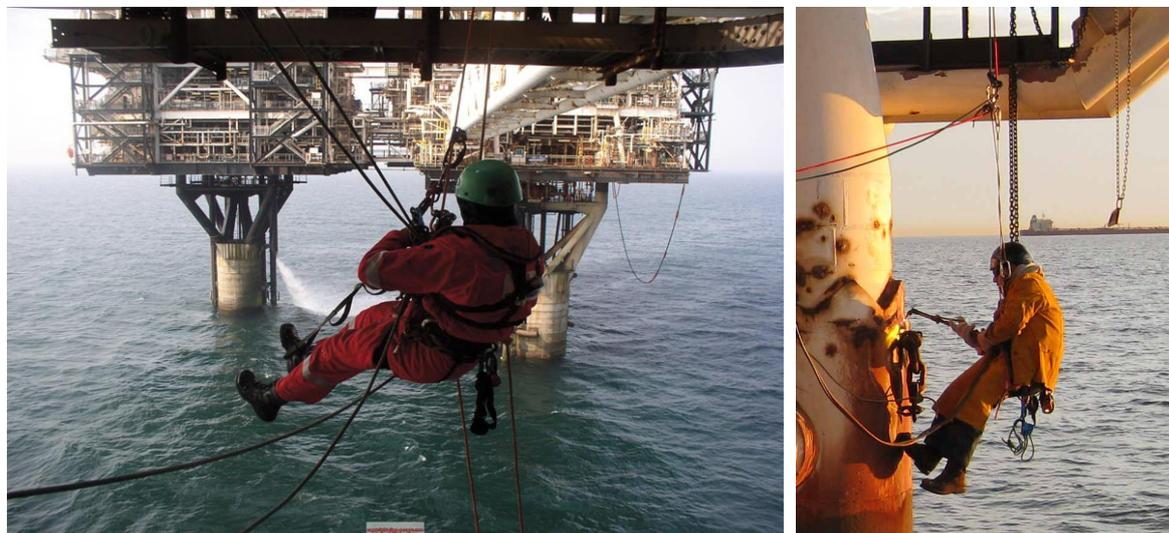
Figure 6.7: Examples of rope-access personnel and welders. (Pictures from *arabianoilandgas.com* and *cecventura.com*)
