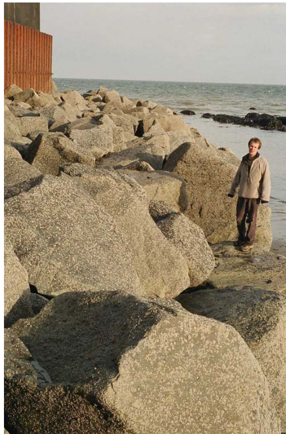
Figure 9: Samphire Hoe: Exposed rock toe at low tide (Courtesy of T Pullen, HR-Wallingford)
