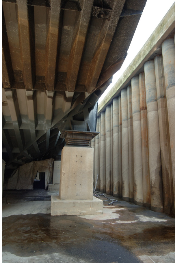
Fig. 2 Compression blocks under the gate at Maeslant Barrier. (Image: Courtesy of Rijkswaterstaat.)
