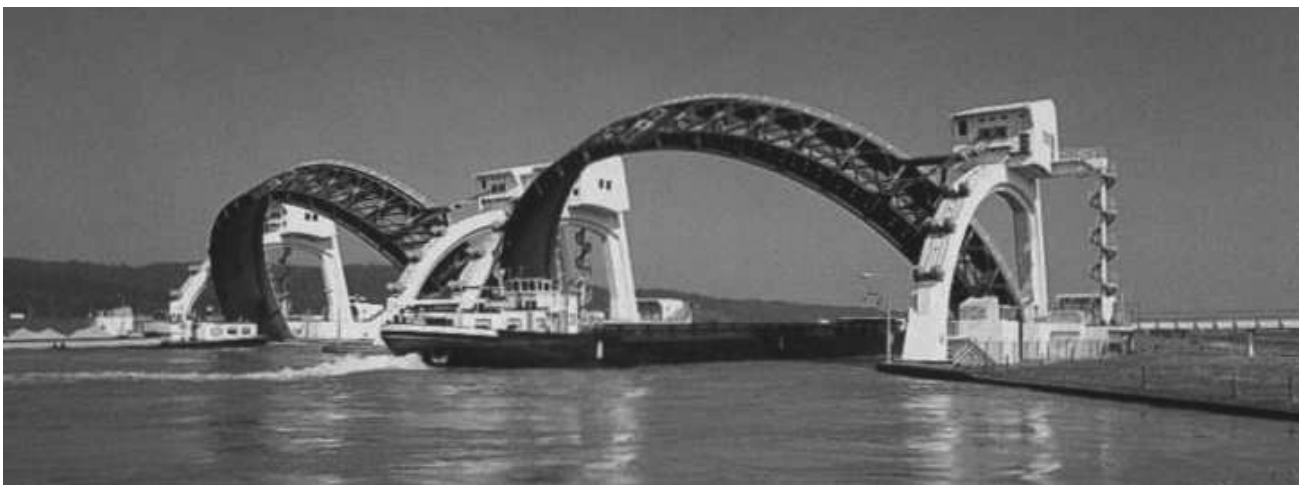
Figure 2-11 Inland barges navigating through opened visor gates, weir river Lek - Driel
