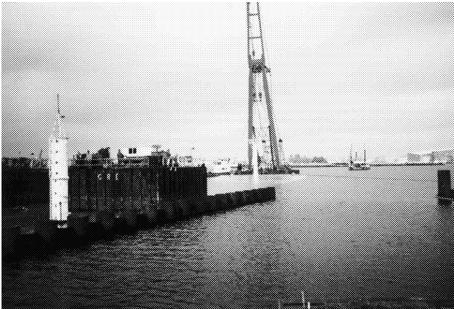
Figure 1-43 Immersed tunnel sections at the Piet-Hein tunnel, Amsterdam
