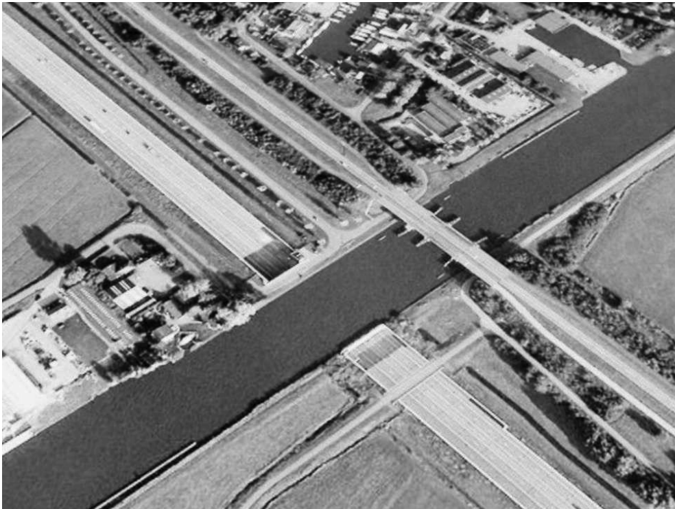
Figure 1-36 Prinses Margriet tunnel with approaches
