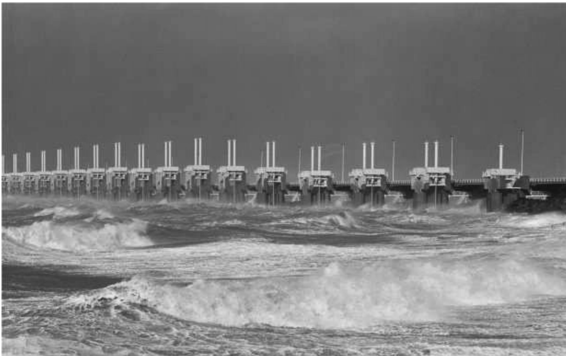
Figure 1-58 Storm-surge barrier in the Oosterschelde
