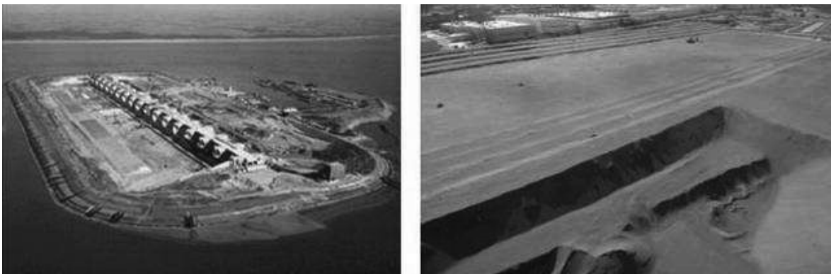
Figure 1-31 Building pit; In the waterway (left), on land (right)
