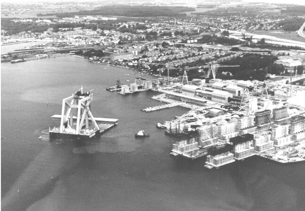
Figure 5-5 Svanen at the prefab-yard, Nyborg, Denmark
