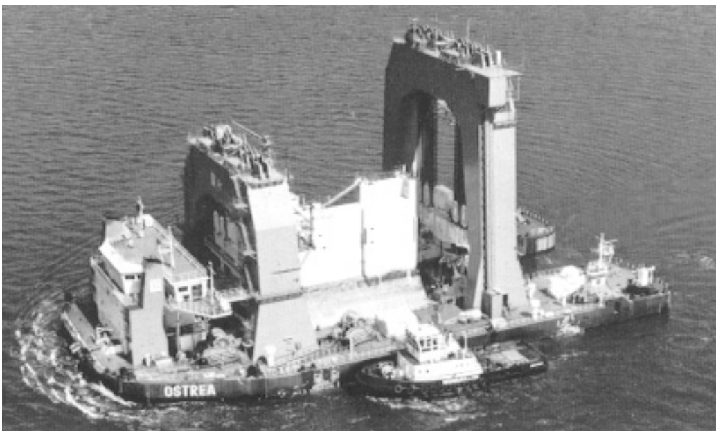
Figure 5-6 Floating crane Ostrea transporting a pier of the Oosterschelde barrier
