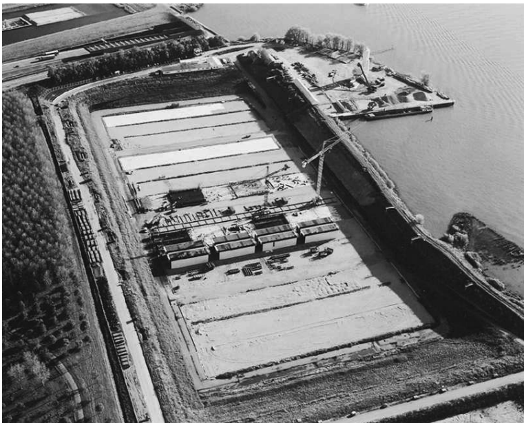
Figure 1-33 Tunnel sections for the HSL railway line in a construction dock
