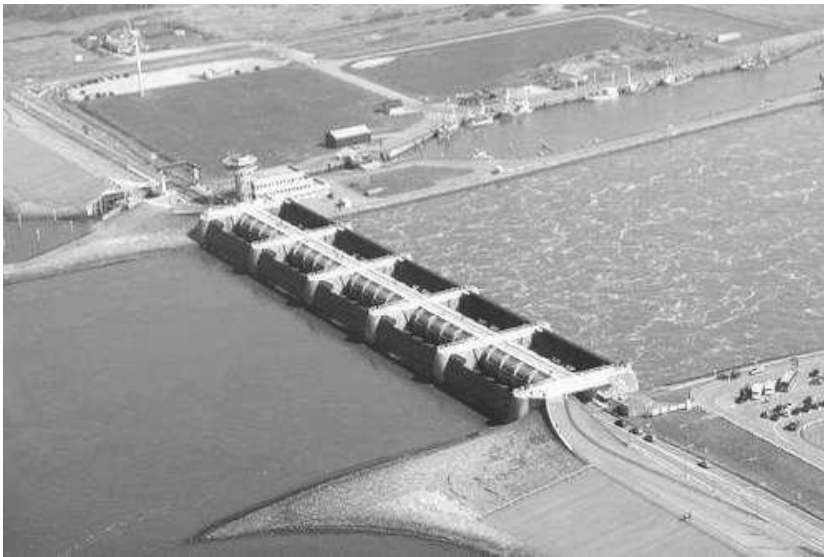
Figure 1-49 Dewatering gate at or in the Eiderdam
