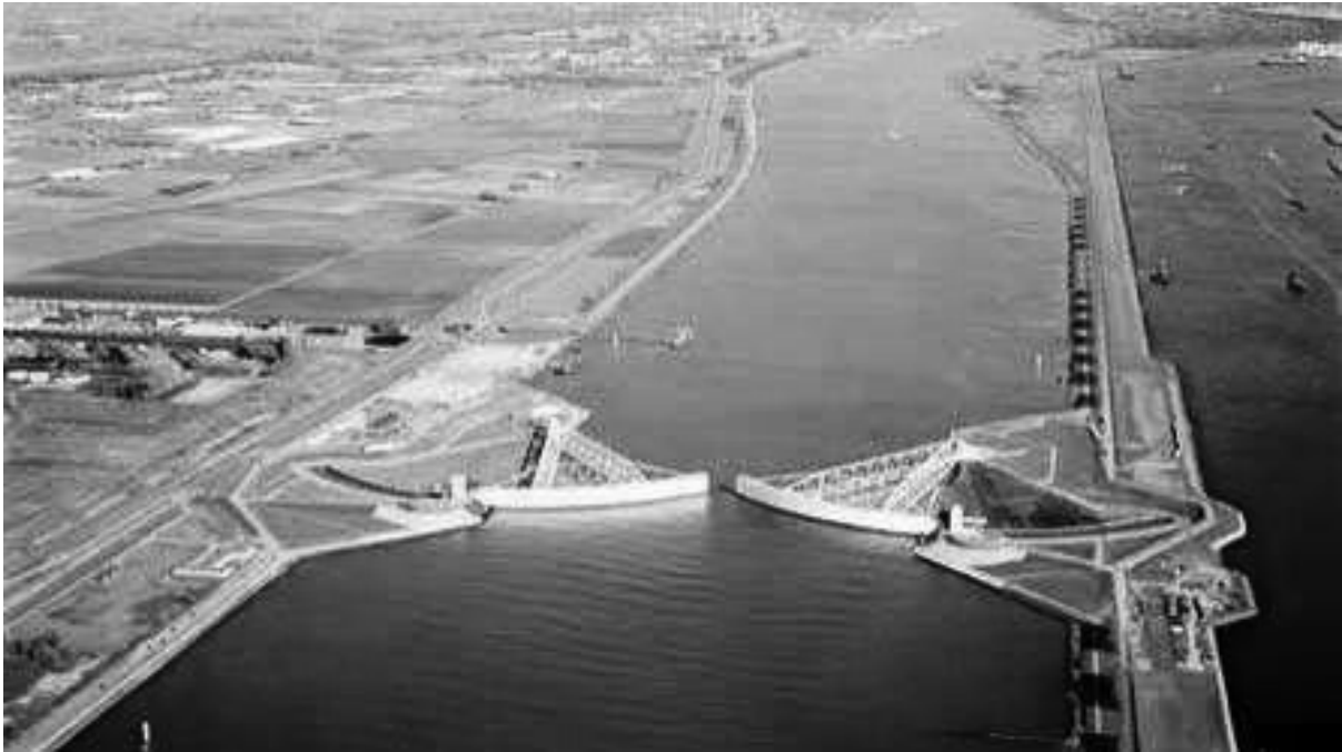
Figure 1-59 Storm-surge barrier in the Nieuwe Waterweg (Maeslantkering)
