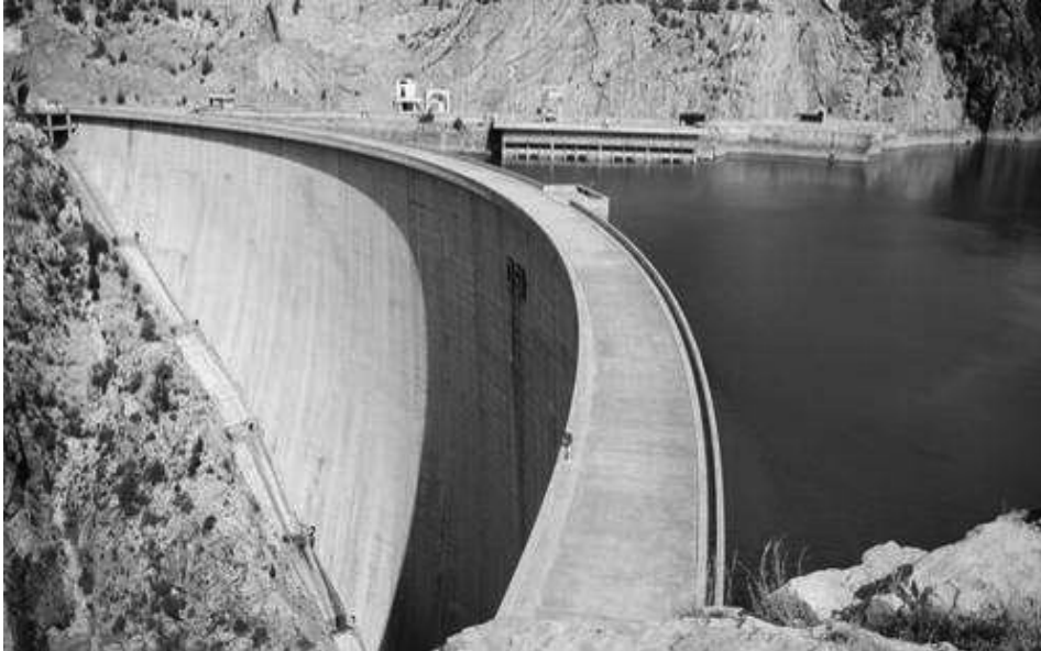
Figure 1-60 Concrete arch dam and spillway
