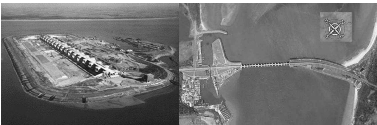
Figure 3-5 Construction pit (period 1958-1968) - left, Overview Haringvlietdam (2005) - right
