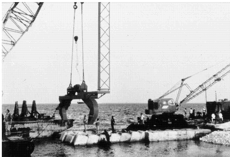
Figure 1-14 Construction of a sloping bond quay wall
