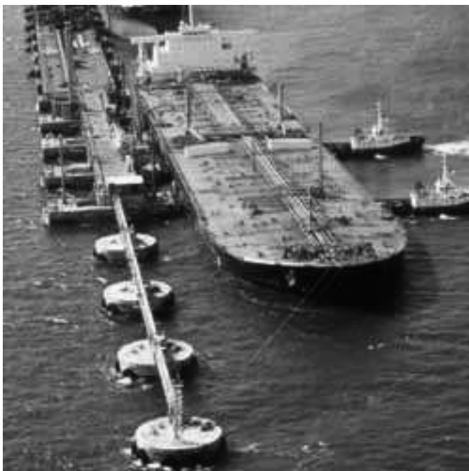
Figure 1-27 Cellular cofferdams used as mooring dolphin
