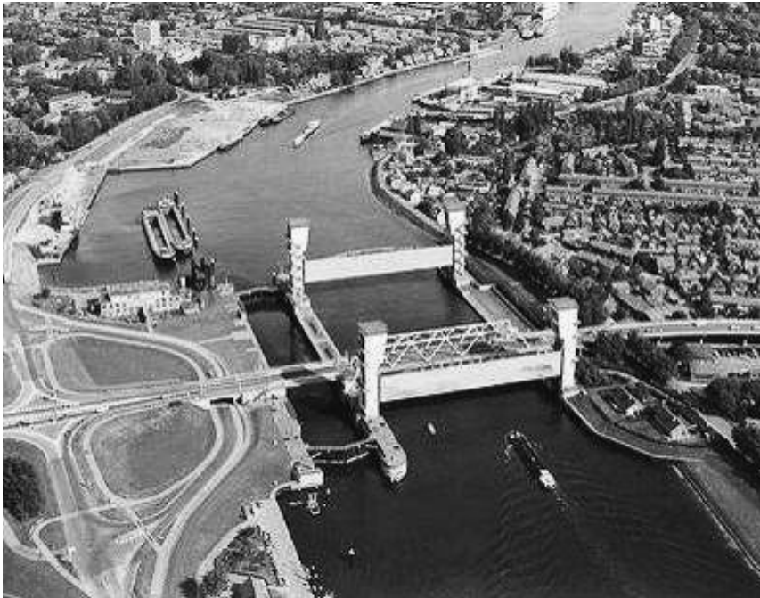
Figure 1-57 Storm-surge barrier near Capelle aan de IJssel
