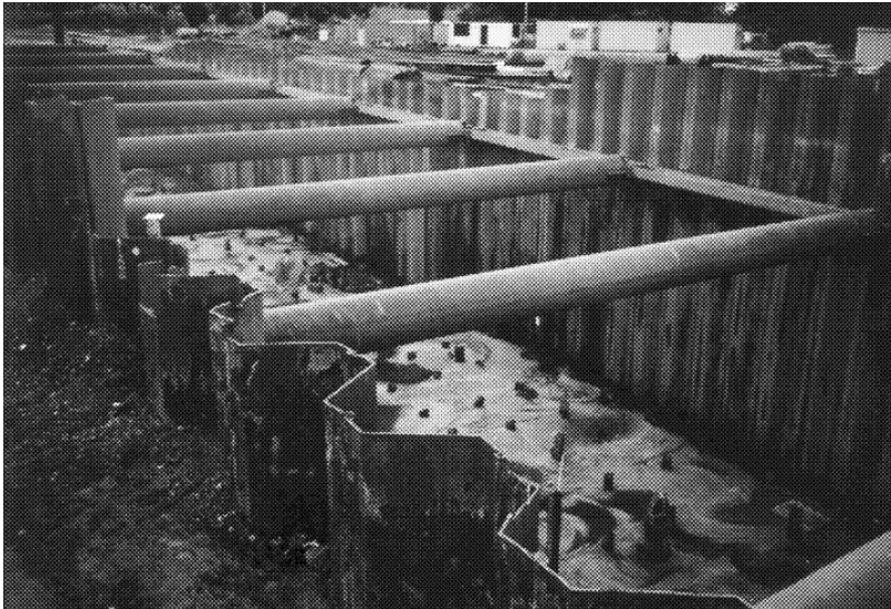
Figure 1-32 Cofferdam or braced excavation
