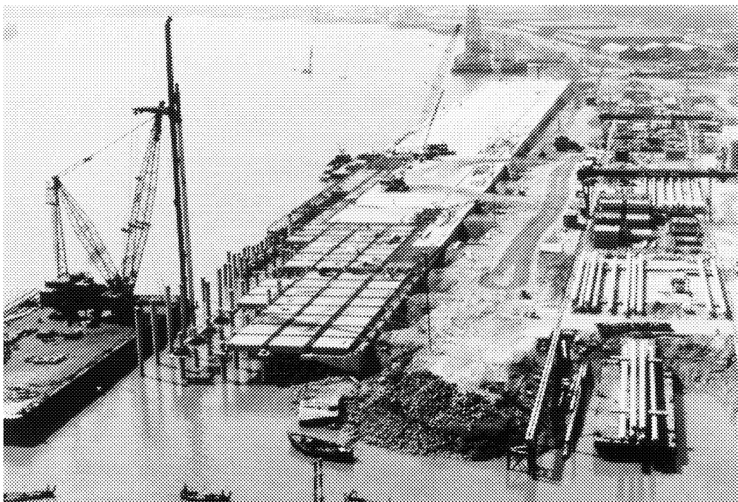
Figure 1-18 Precast platform under construction
