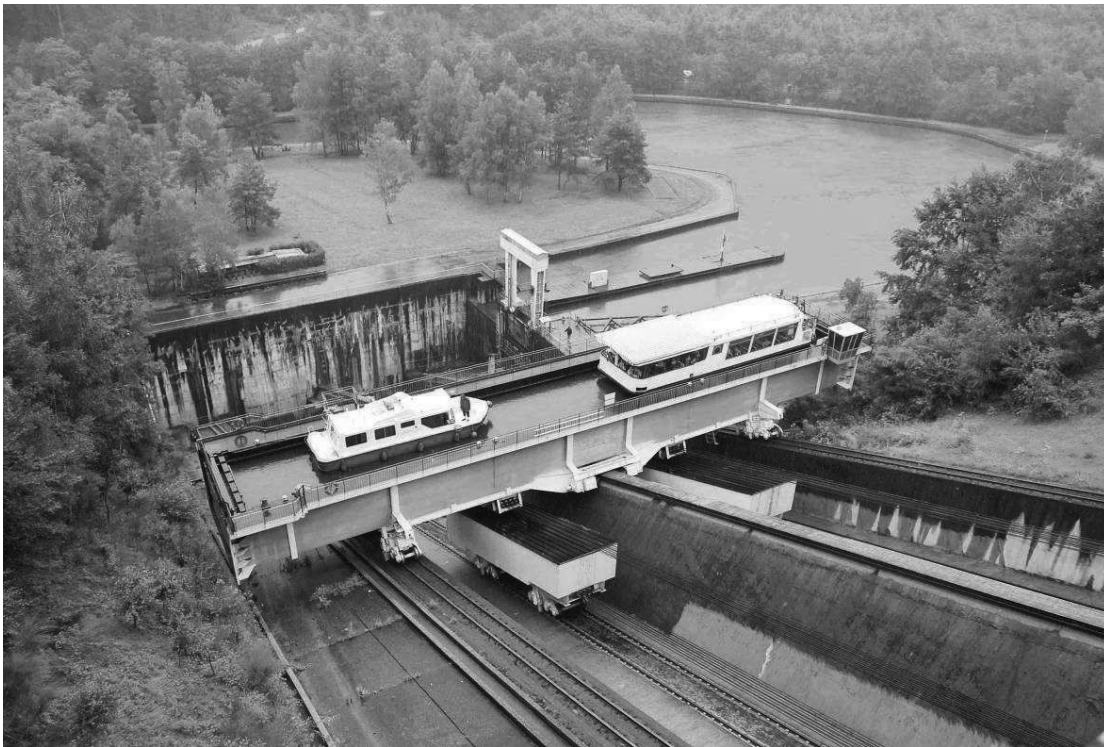
Figure 1-55 Inclined plane in lateral direction
