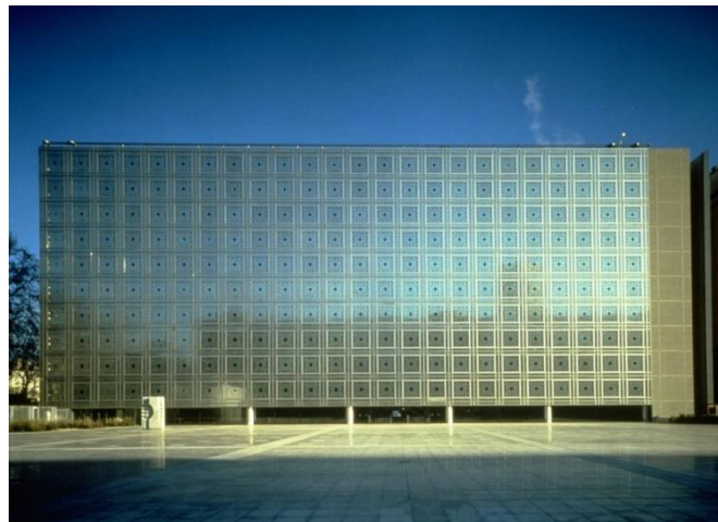
Figure 17: Arab World Institute facade, which features mechanical irises that open and close according to interior light quality. 3
