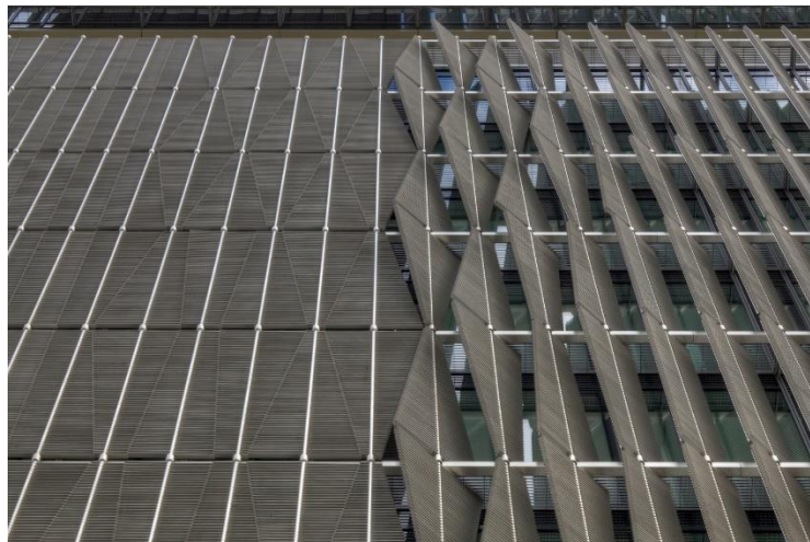
Figure 26: stainless steel lamellas, which track the sun and rotate automatically throughout the day 7
