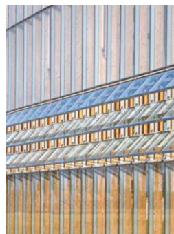
Figure 27: a) The 'glass box' of the academy, b) View of openable vents in the atrium facade
