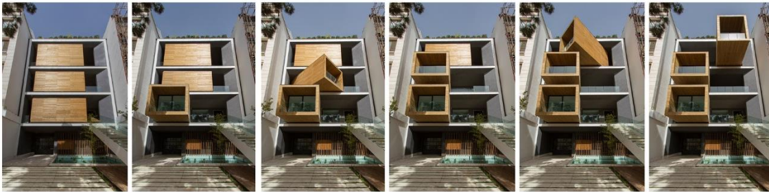
Figure 151: time lapse of rooms of Sharifi-ha House being moved. 51
