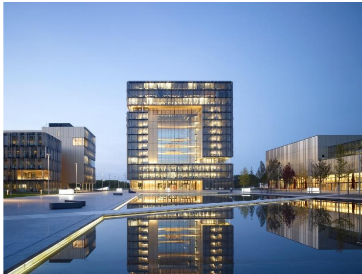
Figure 25: Q1 building on the campus of ThyssenKrupp AG in Essen, Germany 6
