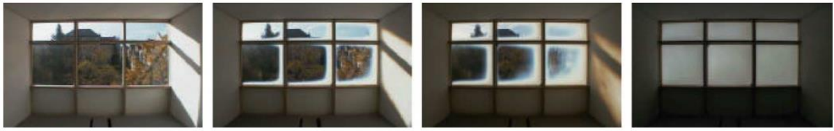
Figure 34: a thermotropic resin used as a window, to provide adaptronic glare and overheating reduction. This example, from (Nitz & Hartwig, 2005), takes 15-60 minutes to activate. Using it on all the windows of a room was not recommended, due to obstruction of views
