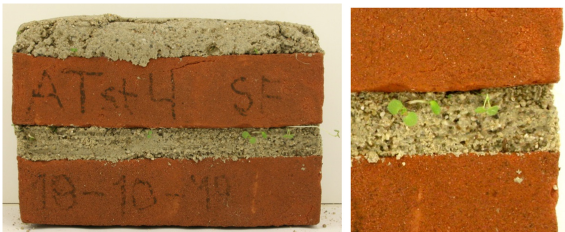
Fig. 11. Plant growth after 3 months outdoor exposure on ATst4-S-B2 specimen.
