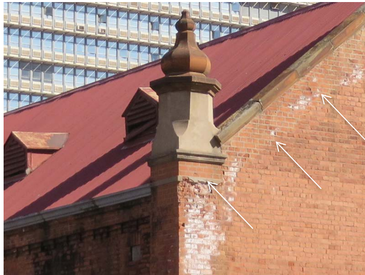
Figure 4: The Old Government Printing Works in Tshwane (1898), constructed of soft brick. The parapets were replaced with an incompatible harder brick in the late 1990s leading to salt efflorescence and disintegration of the softer brick. The line indicating the transition from original to later material is indicated (N. Clarke, 2014, adapted).
