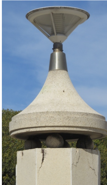
Figure 3: A lamppost at the Sea Point Swimming Baths, Cape Town, attributed to Dutch architect, Jaap Jongens. Spalling, cracking and exposed corroded reinforcement of concrete in a marine environment. This column also exhibits the effect of uninformed maintenance work, especially evidenced by the new pointing (N. Clarke, 2015).
