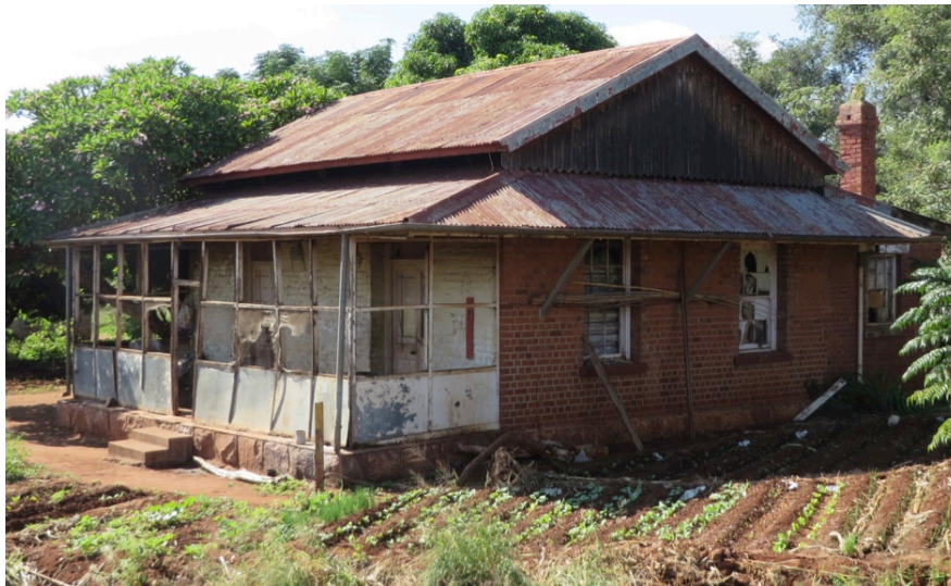
Figure 2: Climate adaptive designed staff housing at Kaapmuiden Station on the NZASM Eastern Line dating to c.1898. The double roof and large overhangs were a response to the hot and humid conditions of the Mpumalanga Lowveld (N. Clarke, 2016).
