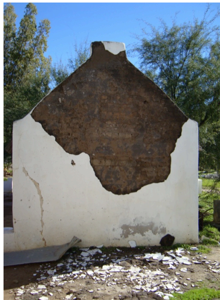
Figure 1: Failure of an uninformed repair project in the historic mission town Wupperthal, South Africa. Soft mud brick construction with later Portland cement plaster leads to façade failure (N. Clarke, 2013).
