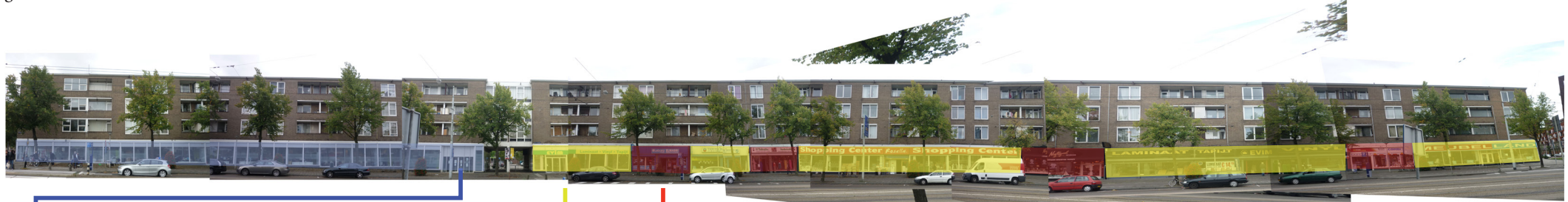
fig 65 Entrances at the commercial street
