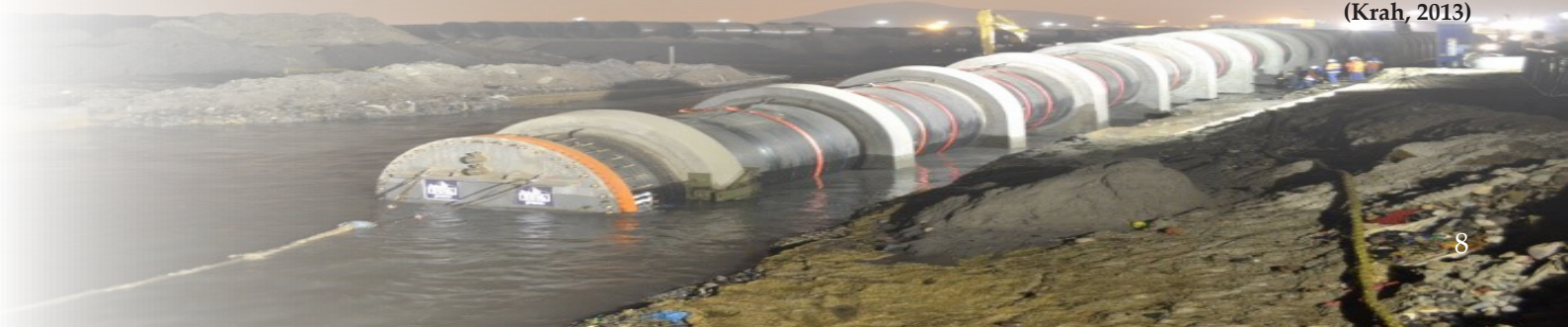
▶ Figure 12: Concrete weights to ballast the HDPE pipe (Krah, 2013)
