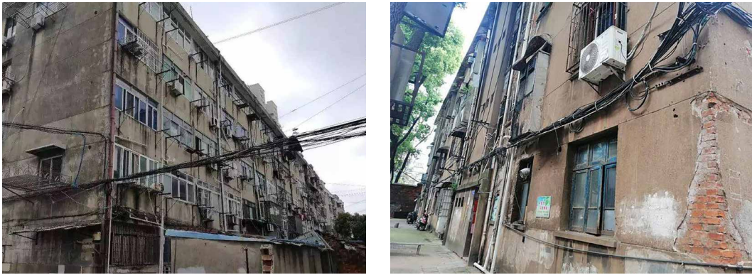
FIG. 1.1 Aging residential buildings
