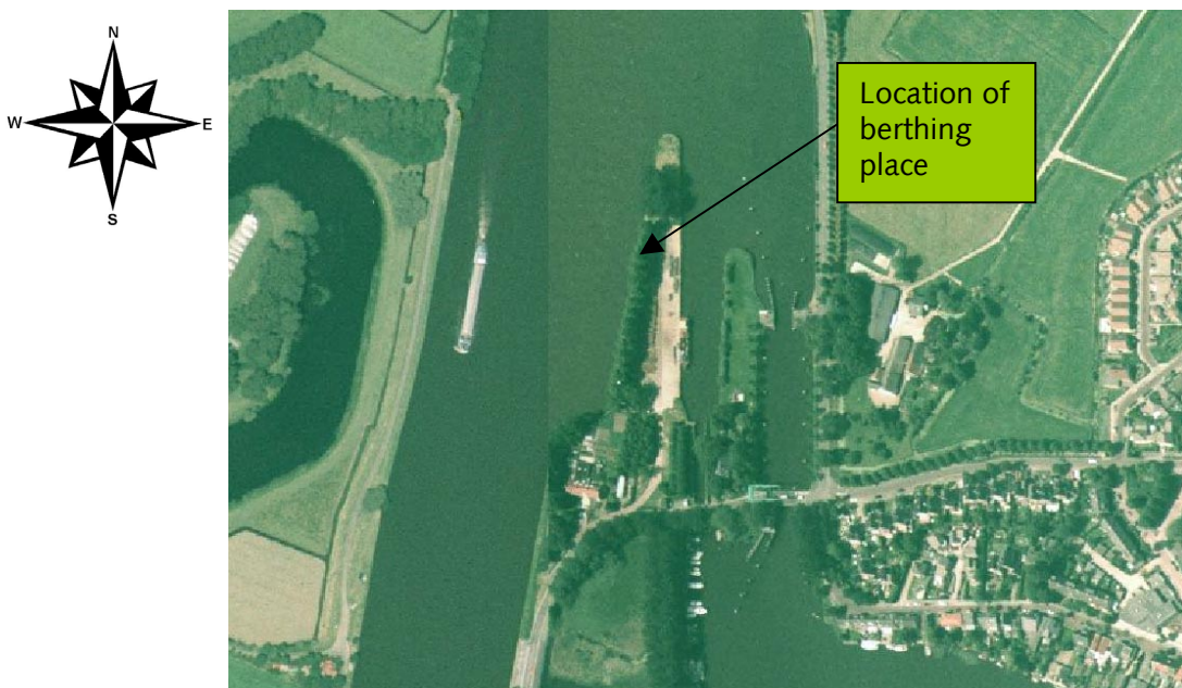
figure 6-12 Aerial photograph of the situation at Nigtevecht.
