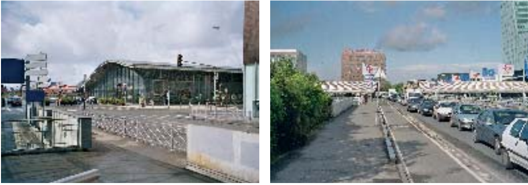
Figure 9.6 The Le Corbusier viaduct crossing the station building, seen from above the ring road (left) and from the inner city towards Lille Europe station (right)
