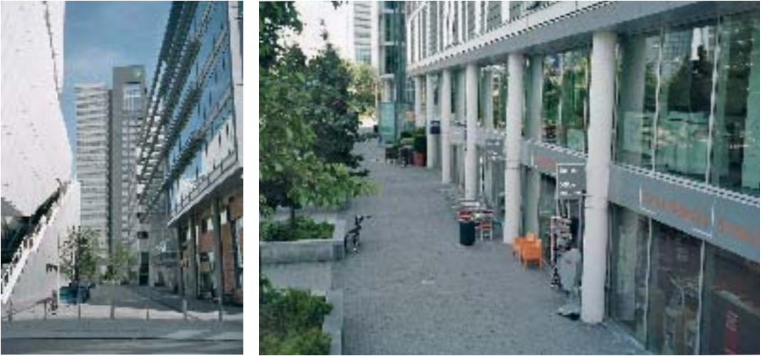
Figure 9.10 Relatively narrow streets and public functions in the plinths of buildings, in the ‘diagonal’ main street of Mahler (left) and, already a more established area, in the WTC at the Zuidplein (right; see also Figure 9.12)
