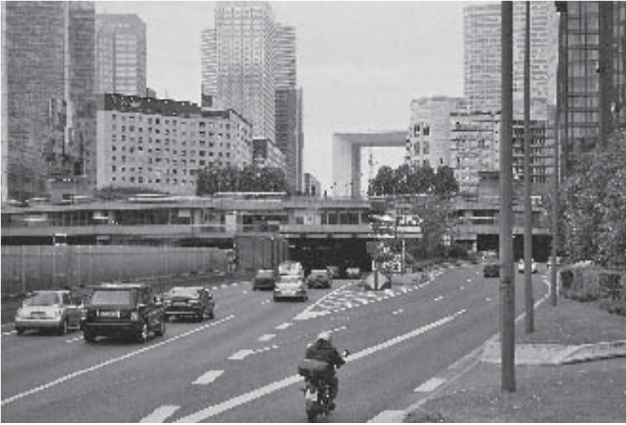
Figure 5.1 Tunnelling may be an effective but expensive way to deal with the negative effects of transport. In La Défense, a 'slab' covers roads, underground car parks and the subway station
