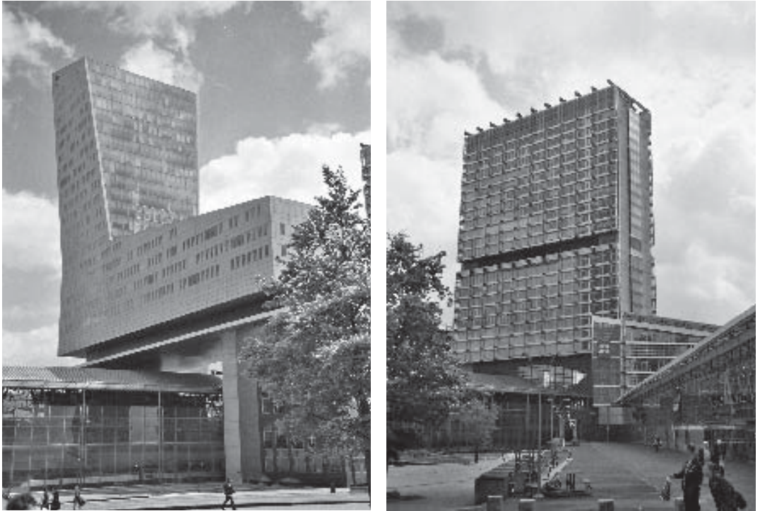
Figure 6.7 The Tour Crédit Lyonnais (Christian de Portzamparc) and the Tour Lille Europe (Claude Vasconi), both built over the railway station
