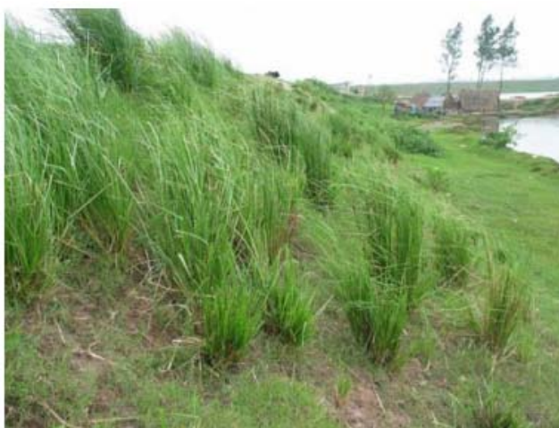
Figure L-15. Types of inner dike slope protection. Left: Vetiver planted on inner dike slope with no structural toe protection. Right: grass planted in grouted stone framework, dike toe is protected by grouted stone longitudinal beam.
