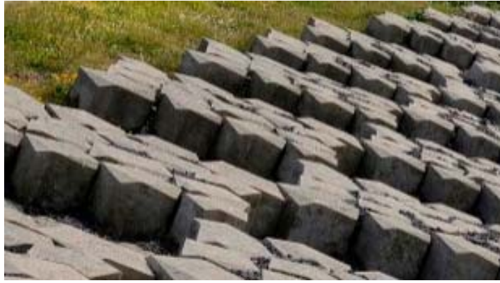
Figure L-14. Discontinuous placement of Basalton® on dike slope
