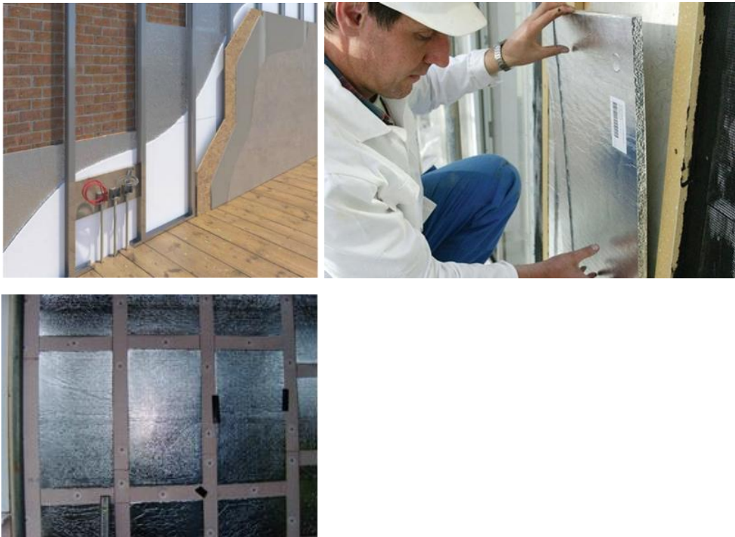
Figure 12 (i) VIP fixing with aluminium channels finished with OSB board. Retrieved from https://www.kevothermal.eu/applications/construction/internal-wall
