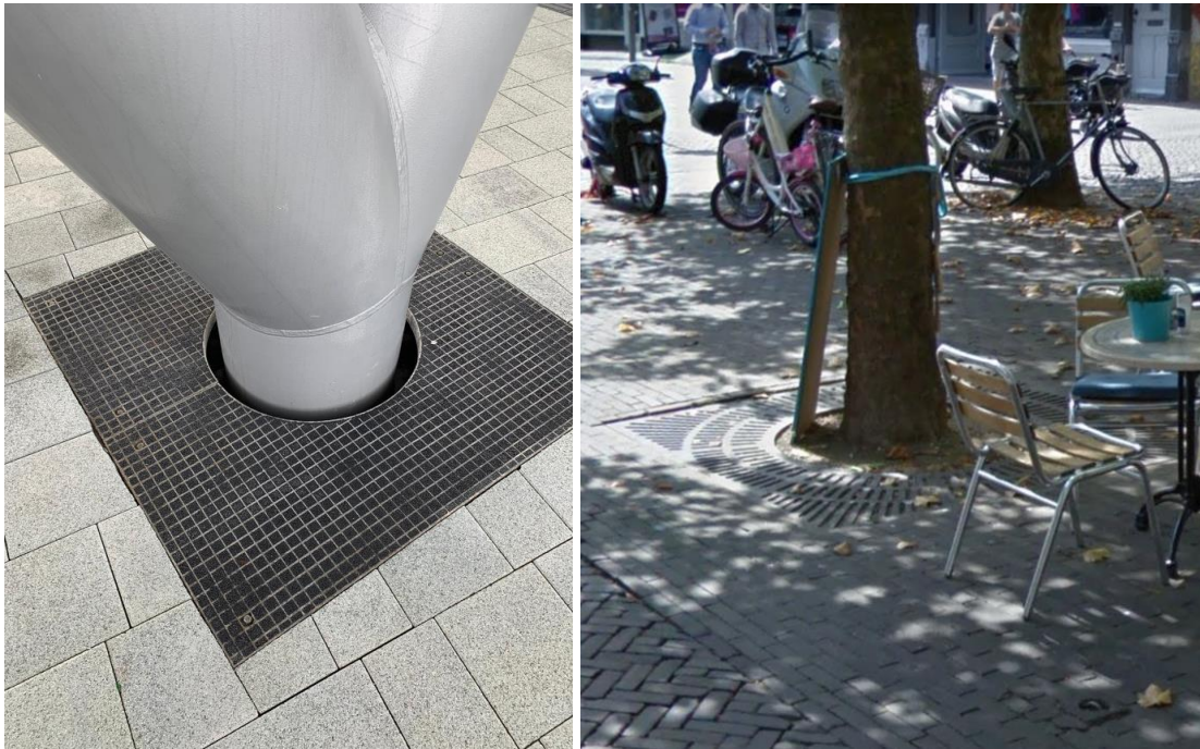
Figure 38 Projects/samples with the same principle with the removable tiles.
