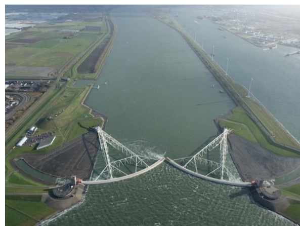
Figure 3: the Maeslant barrier in closed position (Het Keringhuis, 2021)
