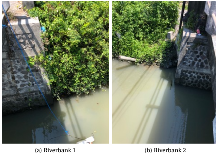
Figure D.2: River banks of the location Pererenan
