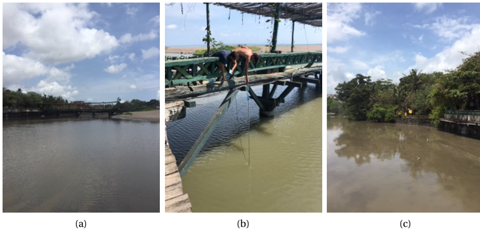
Figure D.6: Photos of the location Berawa
