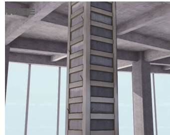
Figure B.9: Jacketing of a column through application of steel plates (Horse construction, n.d.)
