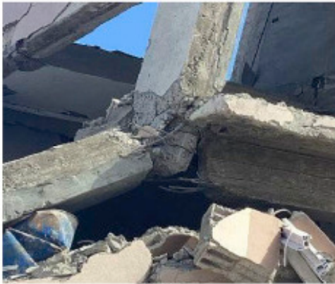
Figure 3.31: Images from the reconnaissance study depicting damage mechanisms to beams (Sezgin et al., 2024)
