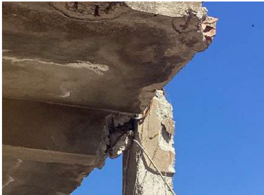
Figure 3.33: Pictures from the reconnaissance study depicting damage mechanisms to member joints (Sezgin et al., 2024)
