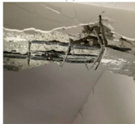
Figure 3.31: Images from the reconnaissance study depicting damage mechanisms to beams (Sezgin et al., 2024)
