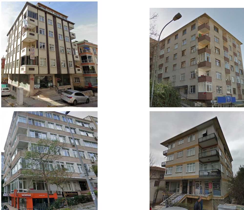
Figure 5.2: Typical mid-rise RC moment-resisting frame apartment buildings in Istanbul: (left top) [Avcılar], (right top) [Üsküdar], (left bottom) [Besiktas], (right bottom) [Kadıköy]. (Google Earth Street View (2014, 2018, 2020, 2025)).
