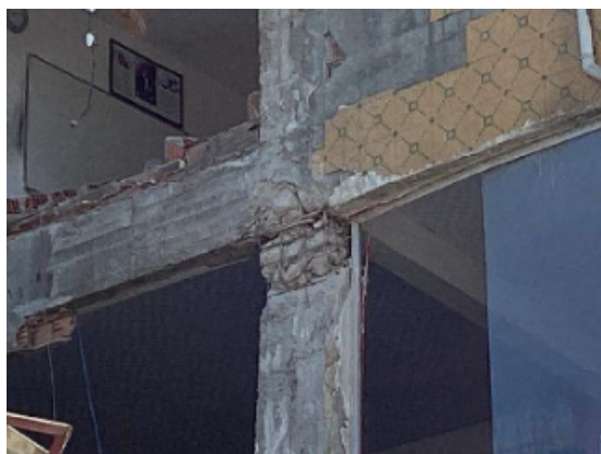
Figure 3.32: Images from the reconnaissance study depicting damage mechanisms to beams (Sezgin et al., 2024)
