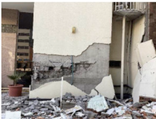
Figure 3.34: Images from the reconnaissance study depicting damage mechanisms to shear walls (Sezgin et al., 2024)
