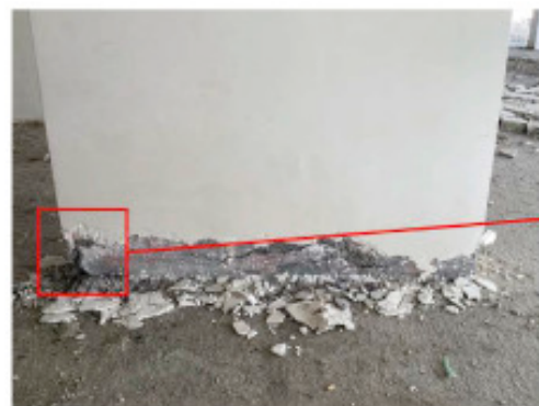
Figure 3.34: Images from the reconnaissance study depicting damage mechanisms to shear walls (Sezgin et al., 2024)
