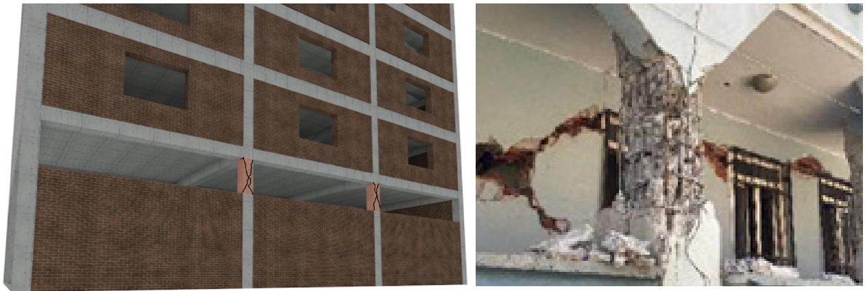
Figure 3.25: The short-column effect illustrated (left; author's own work) and seen in the reconnaissance study (right) (Sezgin et al., 2024)
