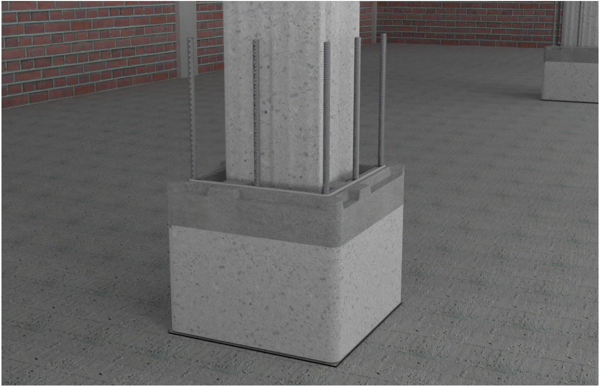
Figure I.7- Step 7: Once the bottom blocks are in place, the first stirrup element is placed in the horizontal grooves of the block elements, in order to confine the system.
