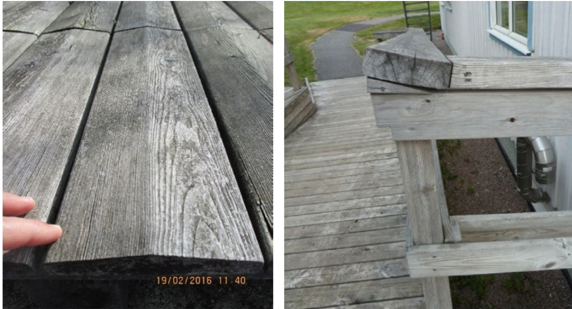
Figure 2.11: Water draining and avoidance of water trapping. Left, decking with good details design to allow dripping rainwater and space between two boards to avoid water accumulations. Right, hand rail in Kristineberg, Sweden: Declined surface but gap between two elements with potential for water trapping. [2]
