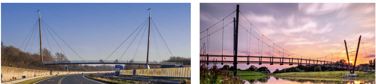
Figure 3.4: Timber cable stayed bridge at Harderwijk for cyclists and pedestrians (left) [20] and a timber suspension footbridge near Arnhem (right) [8].
