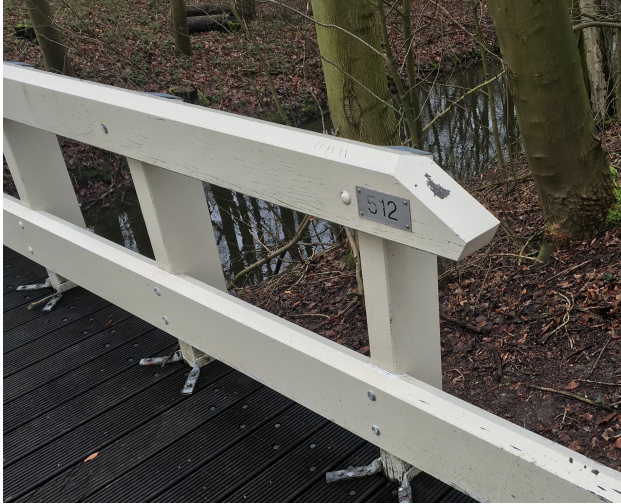
Figure 7.10: Left: Large parts of the railing, covered with a layer of paint, show no visible decay. Right: Longitudinal connection showing paint erosion but no visible sign of decay.
