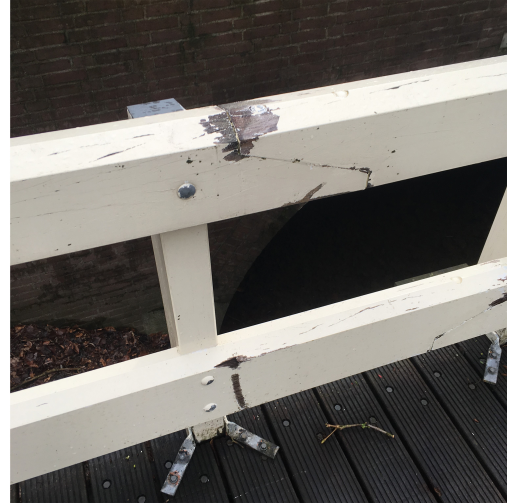
Figure 7.10: Left: Large parts of the railing, covered with a layer of paint, show no visible decay. Right: Longitudinal connection showing paint erosion but no visible sign of decay.
