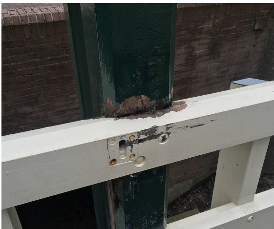
Figure 7.11: At both sides of the fence the connection between fencepost and bridgerailing shows a significant amount of decay.
