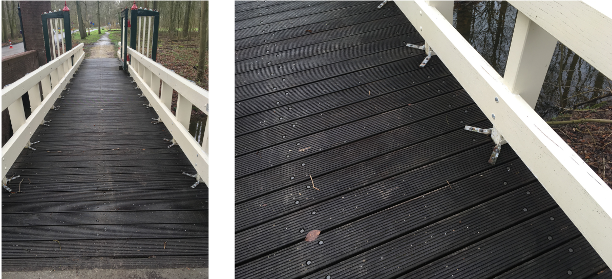
Figure 7.8: The top of the timber deck is still in good condition.
