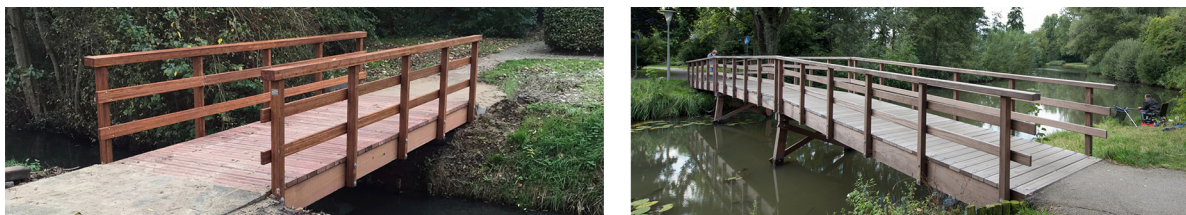
Figure 3.1: Two examples of beam bridges, both located in Arnhem. A single span bridge (left) and a bridge with multiple spans (right) [8].
