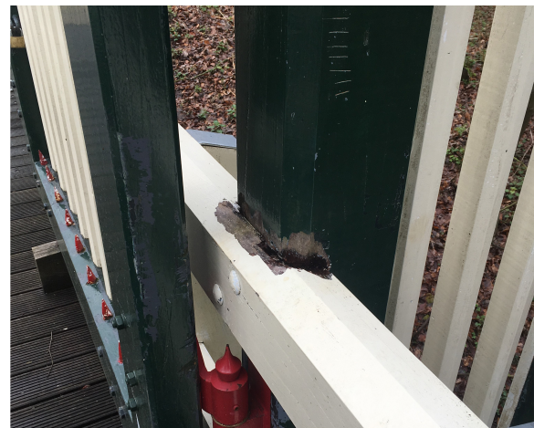
Figure 7.11: At both sides of the fence the connection between fencepost and bridgerailing shows a significant amount of decay.
