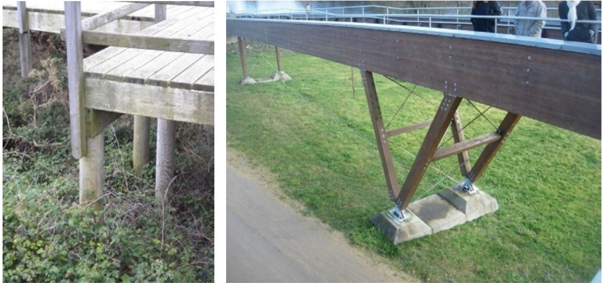
Figure 2.9: Protection from ground contact. Left, pedestrian bridge with pillars in direct contact with ground. Right, pedestrian bridge in Galicia, Spain, with concrete fundamentals and loadbearing pillars separated from the ground. [2]
