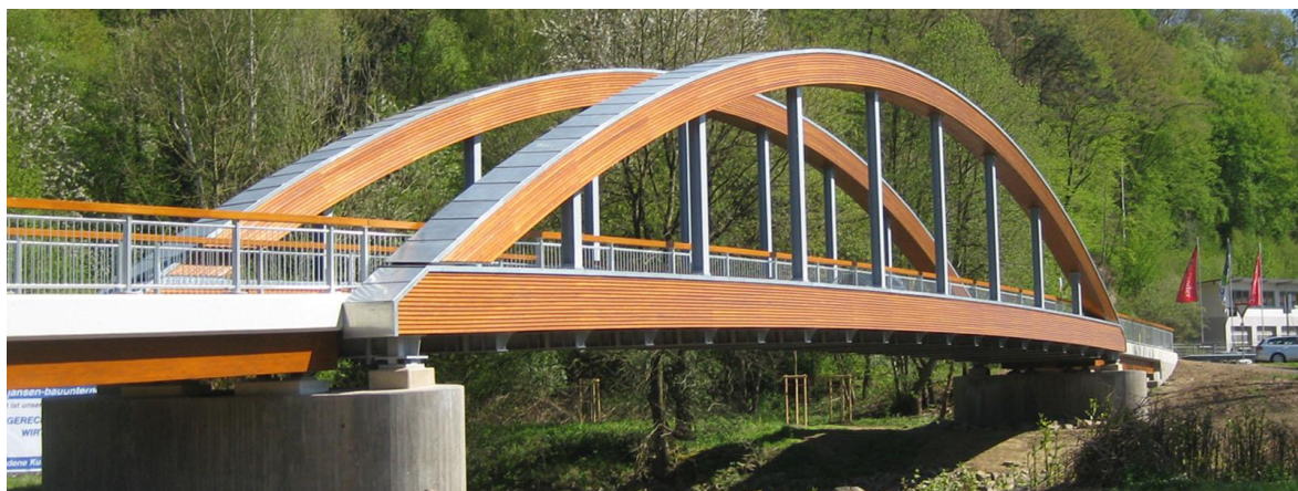
Figure 3.9: Fully protected timber arch bridge located in Lohmar, Germany, build in 2014. The main structural timber elements (arches and main girders made from glue laminated spruce) are protected by titanium zinc covers on top and cladding made from larch on the sides [16]
