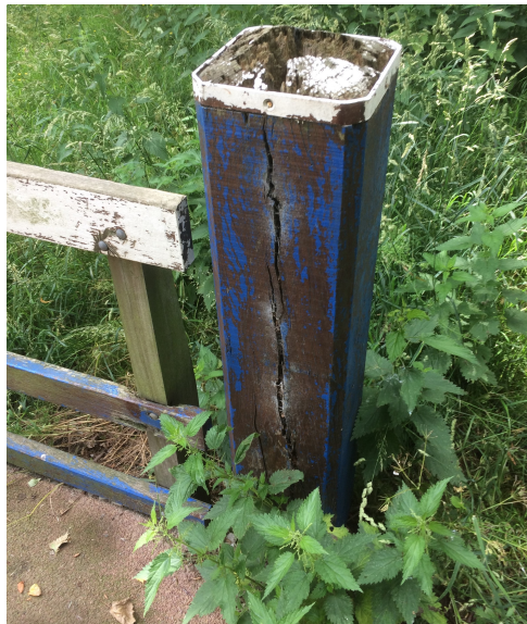
Figure 3.8: Example of vegetation growing around a timber pole
