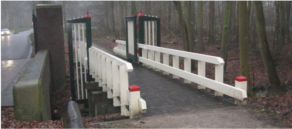
Figure 7.2: Bridge 512 (photo from the Amsterdam database)
