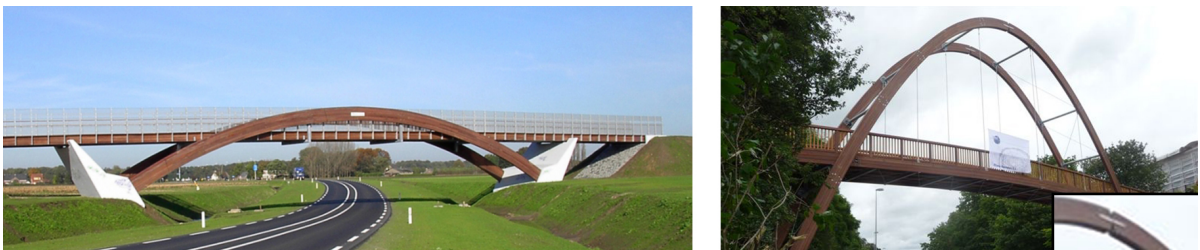
Figure 3.3: A bridge for pedestrians and cyclists consisting of two timber arches crossing the N18 at Lichtenvoorde (left) [8] and a timber arch bridge near Kopenhagen, Denmark (right) [20]. A close look at the connection at the top suggests that this is a three hinged arch.
