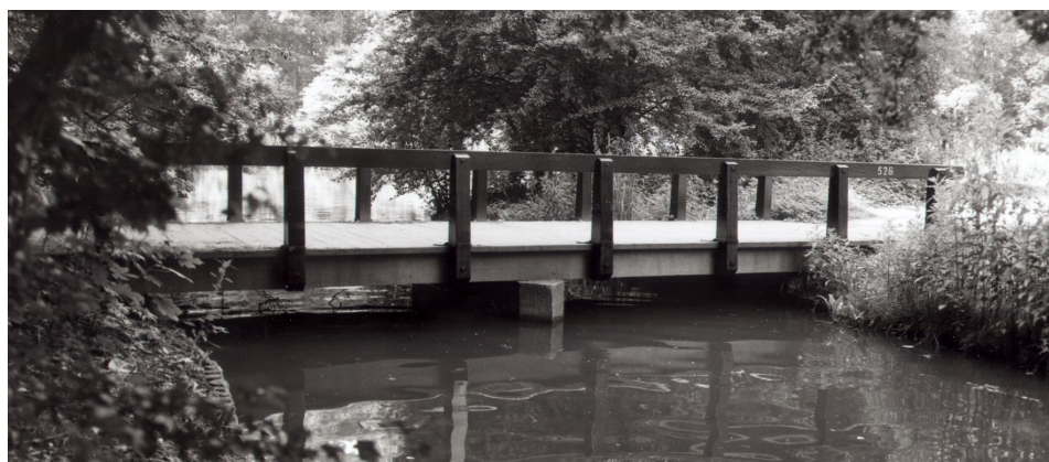
Figure 7.13: Bridge 526 (photo from the Amsterdam database)
