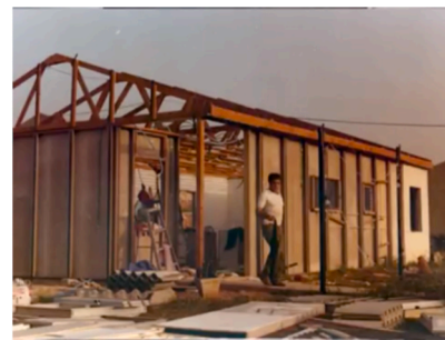
Fig. 3. A temporary house in Mitzpe Sapit. Kochav-Yair Collection.
