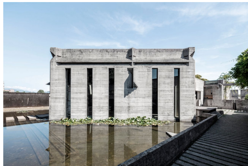
[Figure 2.1.9] (bottom) Brion cemetery, rain-stained concrete from gap in parapet of chapel, photo by author, 2017
