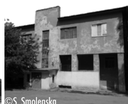
HOUSES FOR EMPLOYEES
