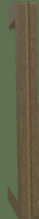
Figure 56: cut in wood for cabling
