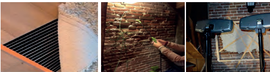
Figure 6: Electric floor heating mats 120 W/m 2 (left); heating wire in joint (middle); infrared patio heaters (right).
