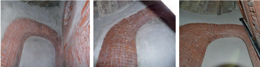
Figure 5: Situation before desalination (left), immediately after desalination (middle) and after 10 years after desalination (right).
