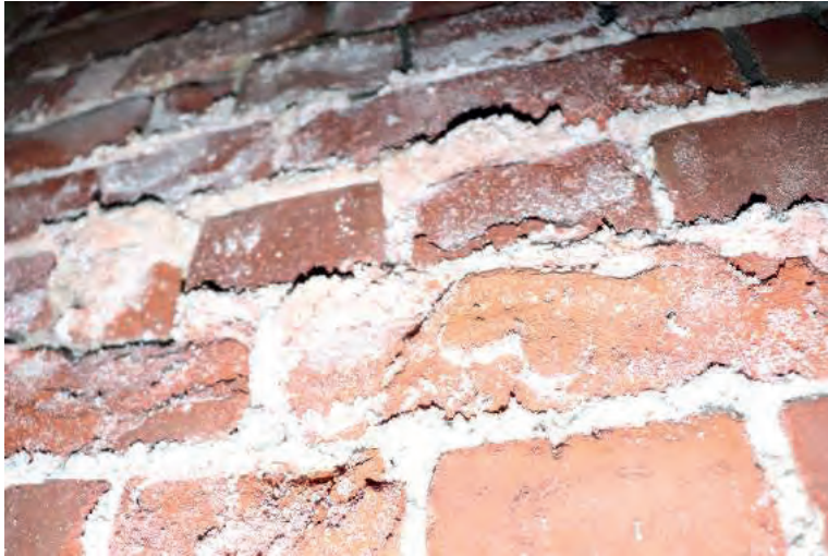
Figure 2: Brick surfaces and salt at the south side of the brick chimney in October 2019
