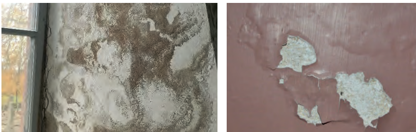
Figure 2: Typical salt related problems in a Neo-Gothic brick church where sodium sulphate is present. Left: Salt precipitation on the surface. Right: Flaking of paint.
