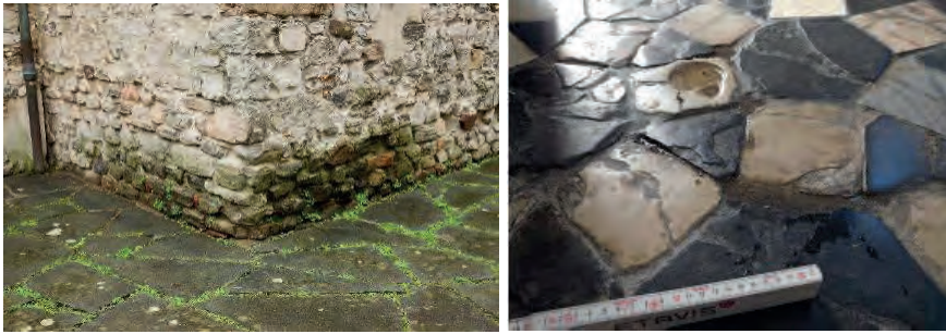
Figure 2: a) Phenomenon of capillary rising damp along the perimeter and biological colonization; b) Puddles of rainwater formed following water entry from the main door during heavy rains.
