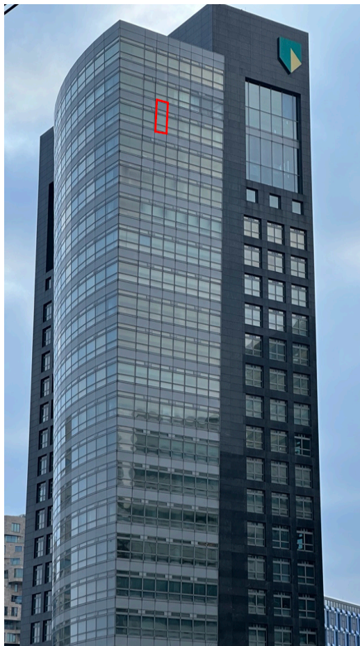
Figure 31: Facade of ABN Amro building (image by author).
