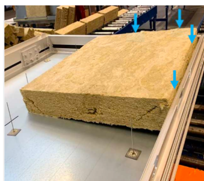
Figure 74: placing insulation on metal pins (image by Scheldebouw).
