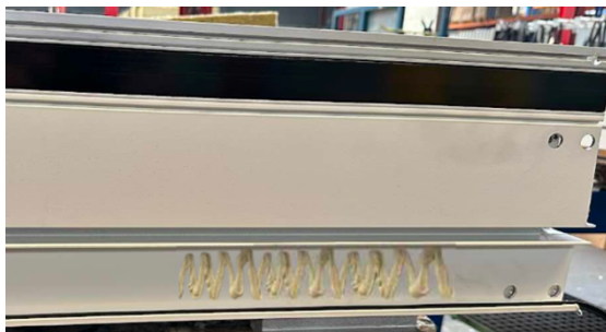
Figure 85: applying non-combustible glue on mullion (image by Scheldebouw).
