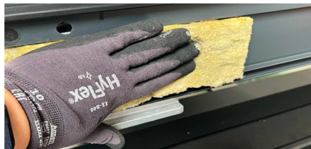
Figure 86: Placing floor stop insulation (image by Scheldebouw).
