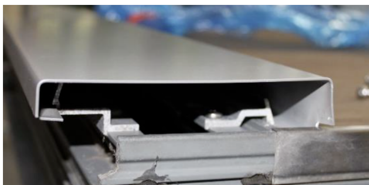
Figure 87: example of aluminum cover cap connected by using snap-fit principle (image by Scheldebouw).
