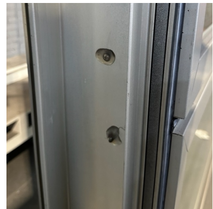
Figure 71: Sealant on screws mullions-transoms (image by author).
