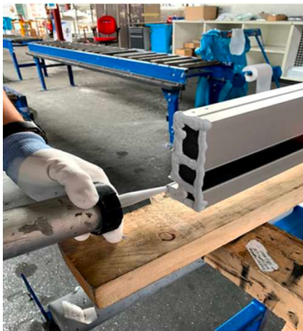
Figure 59: Applying Silicone Sealant on top side of aluminum profile (image by Scheldebouw).
