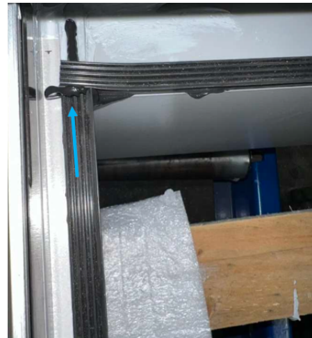
Figure 76: EPDM gaskets placed in aluminum profile (image by Scheldebouw).
