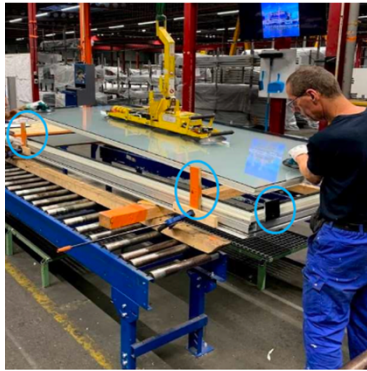
Figure 79: Placing of IGU (image by Scheldebouw).
