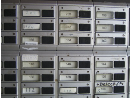
Figuur 4.4-l defect bellenbord
