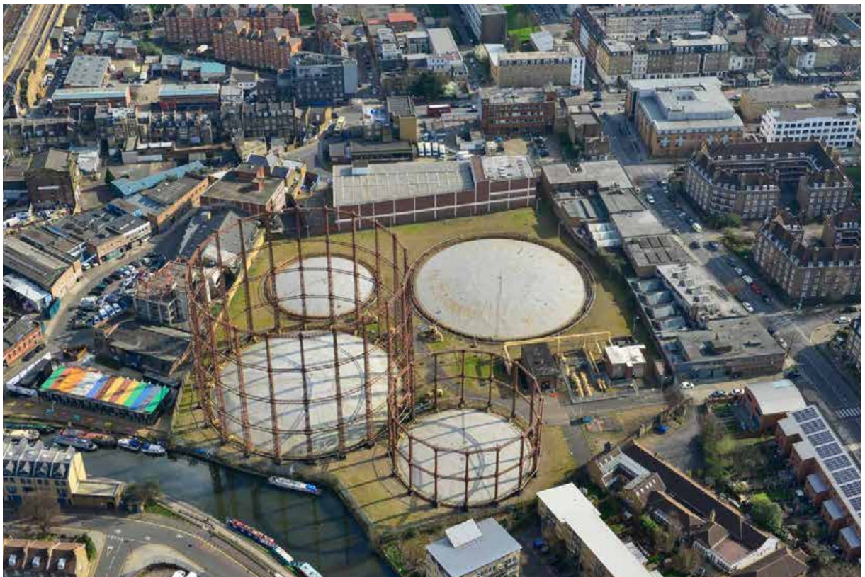
figure 11. Aerial Bethnal Green [Montagu Evans, 2020]
