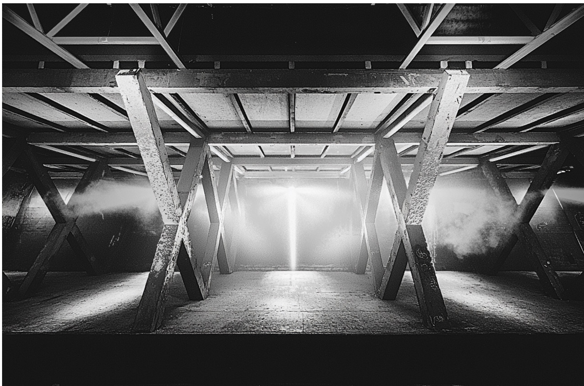
view looking into the cross columns
