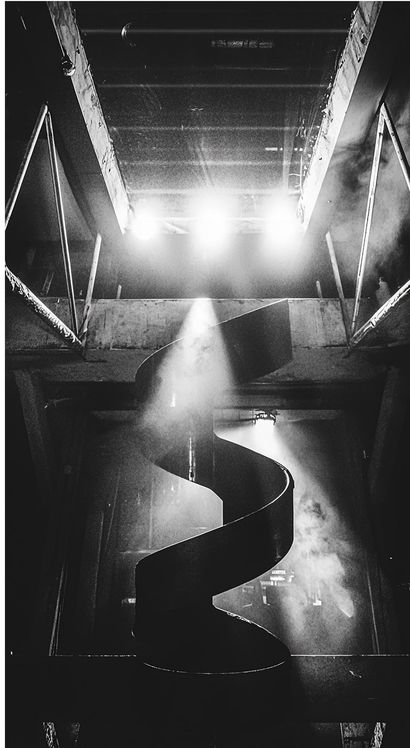
a view showcasing the relationship between the trusses and spiral staircase
