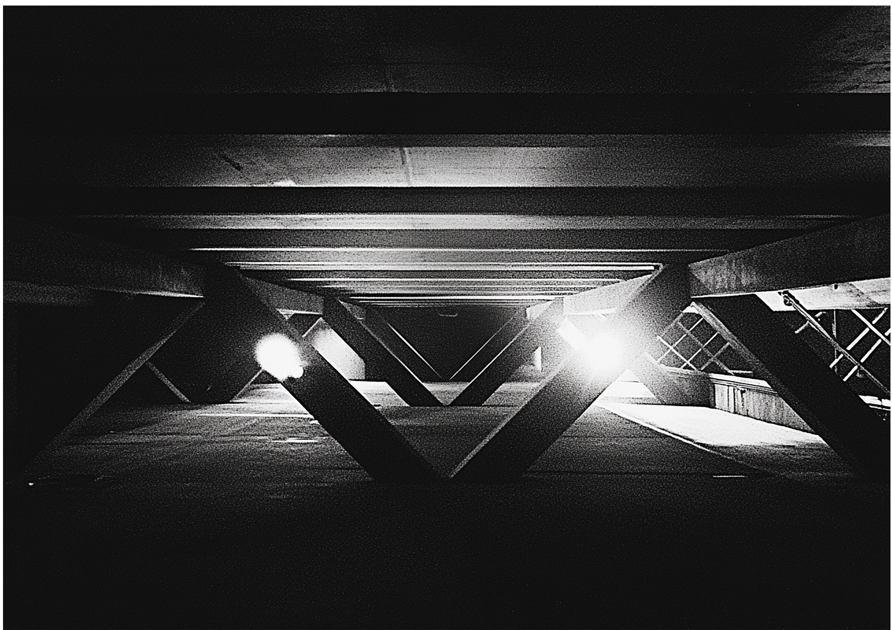
interior view from the second floor
