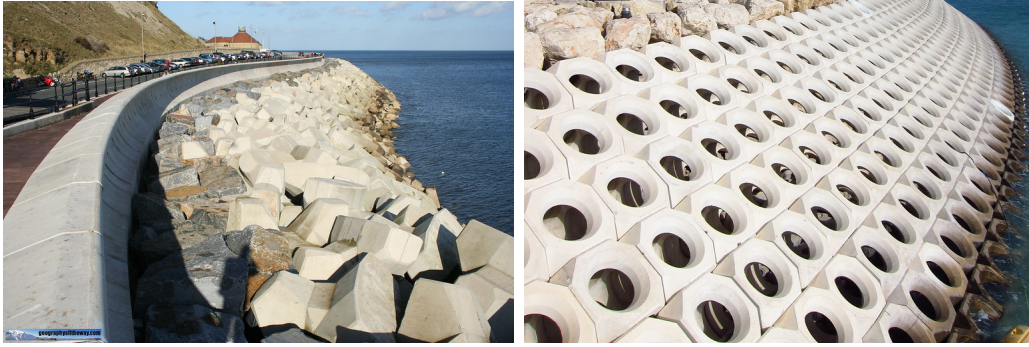
(a) Rubble mound armour with Xbloc (Allaway, 2011). (b) Placed block revetment with Shed concrete armour (Reedijk and Muttray, 2009).
