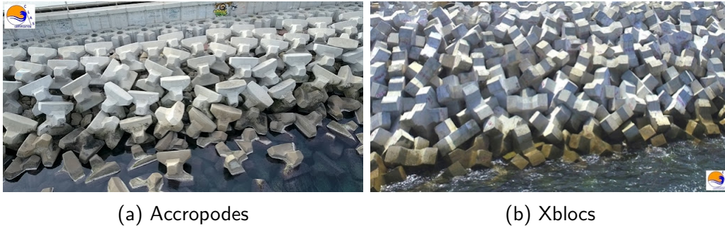
Figure A.6: Different types of single-layer concrete armour units (CLAS Certification, 2018).
