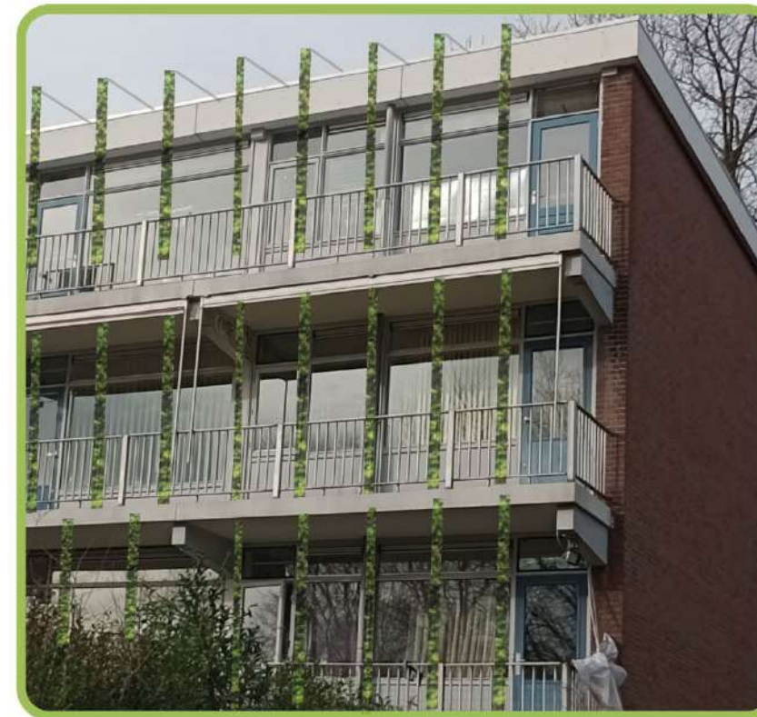
Indirect GF on balconies
