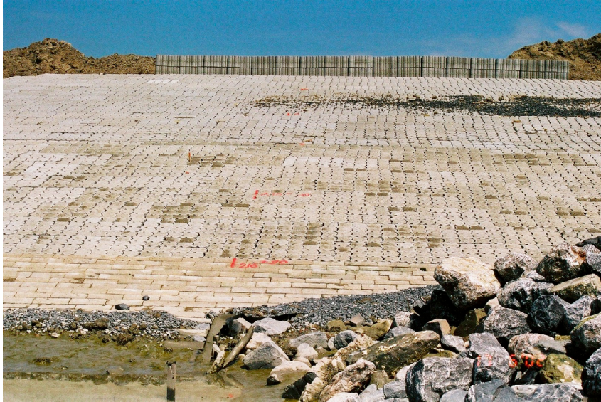
Figure 18: Illustration of the stone pitching (Vrijling 2009)
