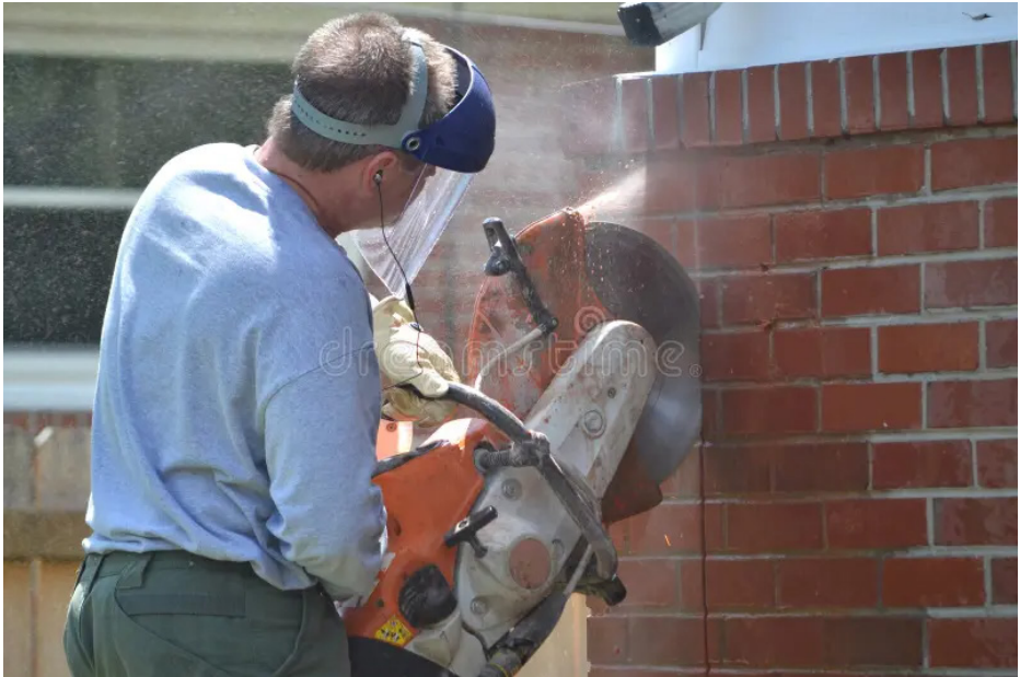
Wall-saw to cut through masonry
