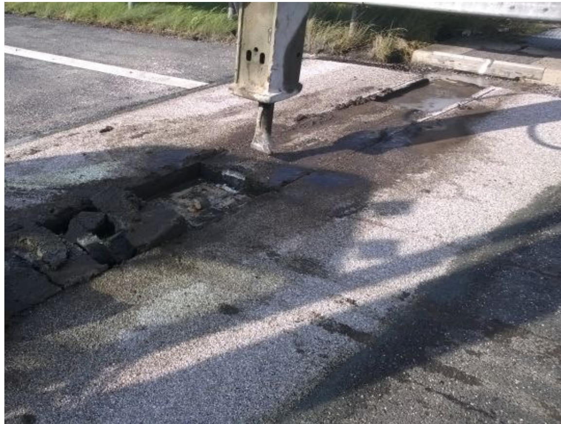
Breaking open the tarmac using a jackhammer, cold planer and excavator
