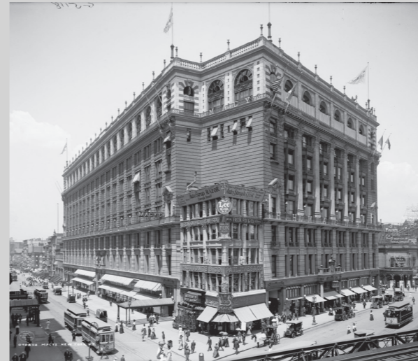
Fig 1- The flagship Macy’s store, on New York’s Herald
