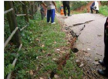
Figure C.2: Horizontal stresses with cracks in the soil (Verruijt and Van Baars, 2007)
