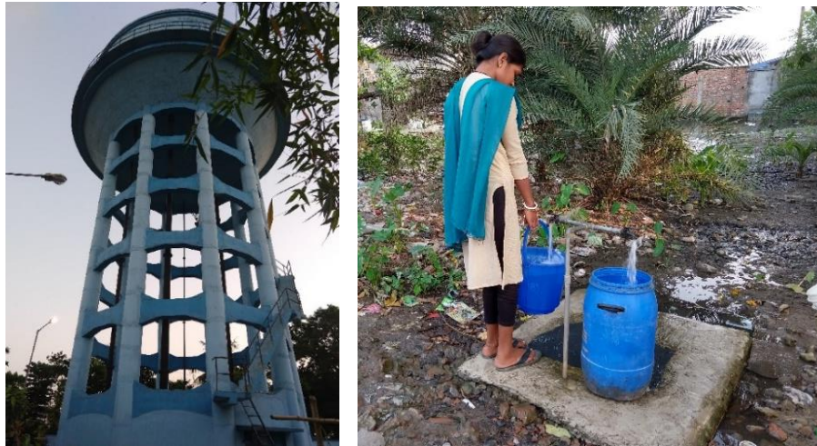
Figure 4.4: PHED drinking water supply – extraction and storage (L) Local distribution via standposts (R)
