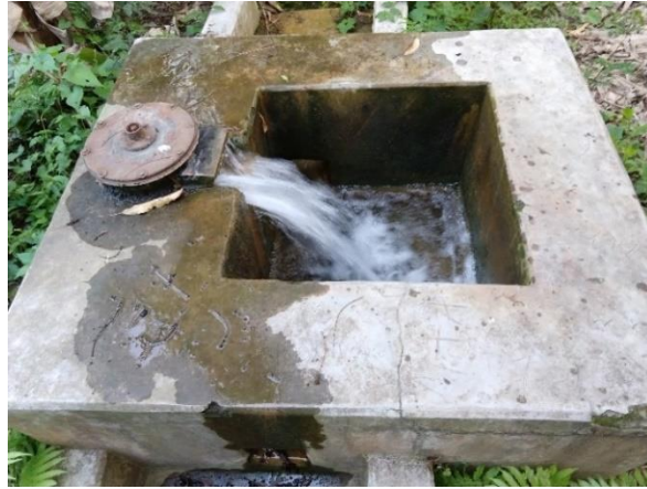
Figure 4.6: End-point delivery of water from irrigation DTW.
