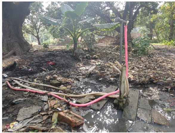
Figure 5.4: Private stand-posts installed in Badai
