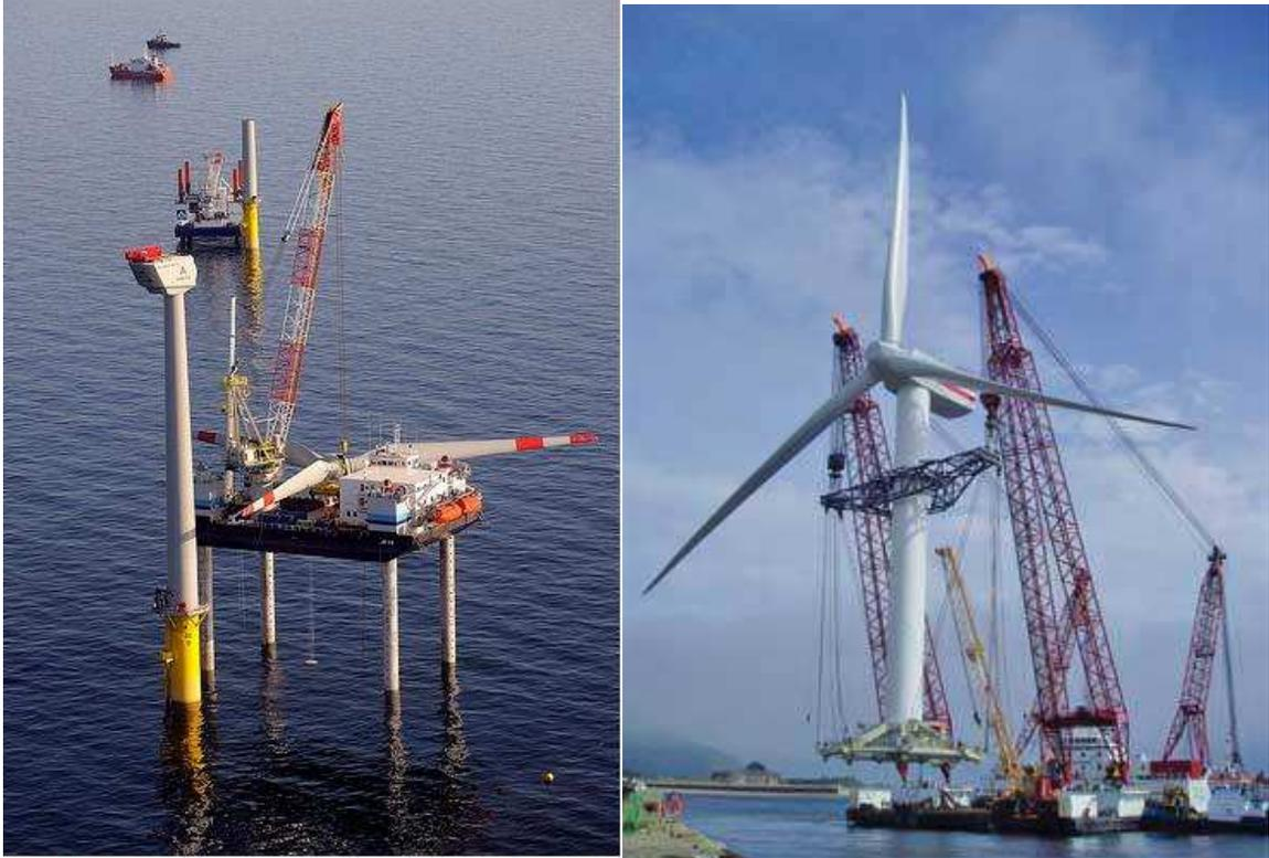
Figure 7-17: Installation with rotor fully assembled (Left). Installation with the wind turbine fully assembled (Right).
