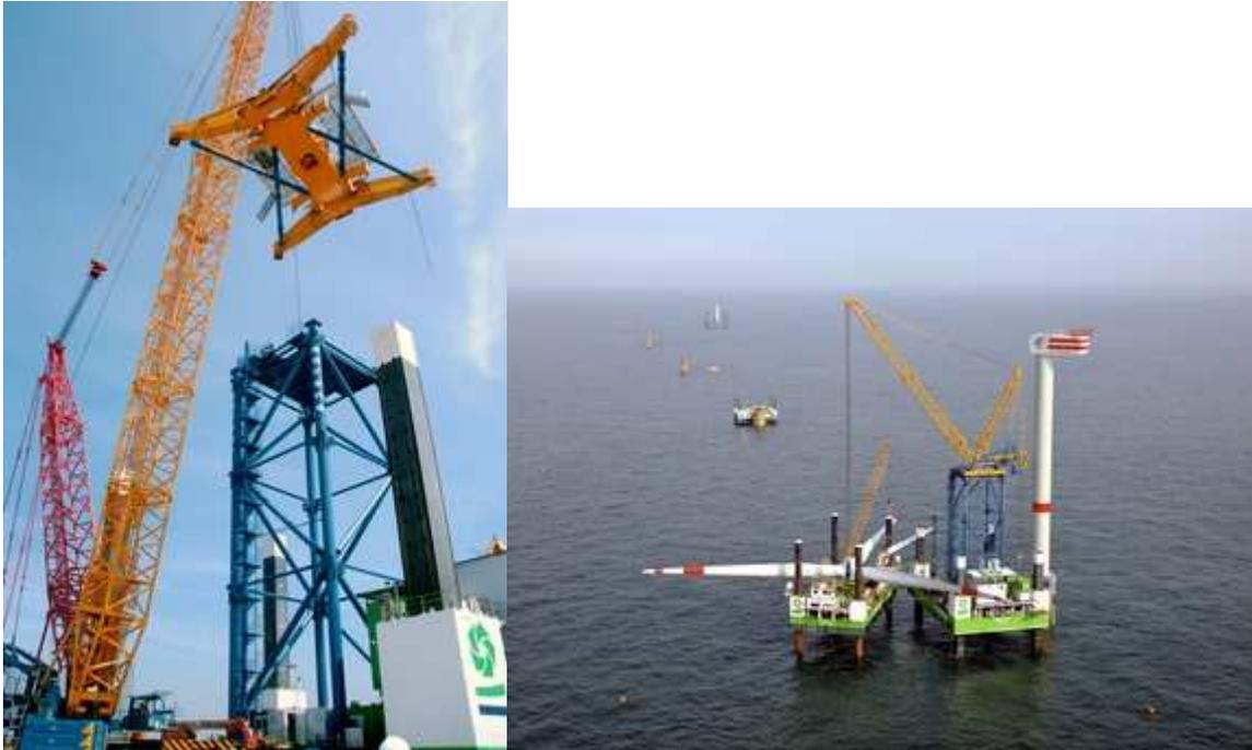
Figure 5-4: Turbine installation at the Thornton Bank wind farm using the modified Buzzard
