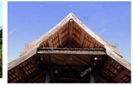
3. Roof space: Served as a insulation layer between the interior and the scorching sun. And
