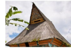
1. Thermal insulation: The Roof is made of thick low thermal capacity materials such as thatches, which gives good insulation against solar radiation.
