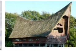
2. Steep Roof: The main purpose of the huge degree of the roof might be the heavy precipitation during raining seasons.
