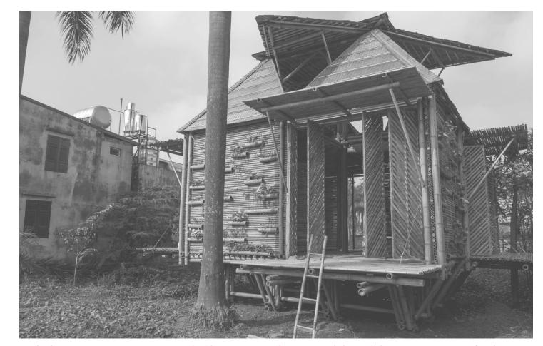
$\parallel \triangleright$  Fig 3 - From the bamboo module of f8-f10cm & f4-f5cm diameter and 3.3m or 6.6 length, each house is simply assembled with bolting, binding, hanging, placing... This pulled monolithic architecture is strong enough to suffer from phenomena like 1.5m-high flood
