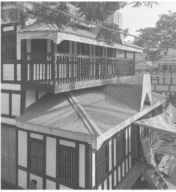
$\parallel \triangleright$  Fig 1/2 - The floor plan tends to be simple and open, which allows for easy reconfiguration to accommodate the changing needs of the household. The construction system is modular, so adding or subdividing rooms is comparatively easy
