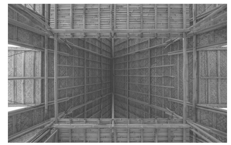
$\parallel \triangleright$  Fig 3 - The house is covered (outside) and partitioned (inside) with light materials (compressed weaved bamboo sheets, leaves, corrugated iron, bamboo screens, etc.) and has a large roof to collect rainwater and harness solar energy. The door systems that can open and close flexibly helps make the house sturdy enough in adverse weather events while creating a typical identity
