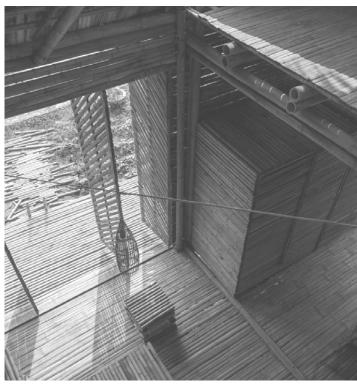
Fig 1/2 - The users can build the house by themselves in 25 days. Besides, it can be mass produced with modules and the total cost of the house is only 2500\$. Therefore, the house can warm people in the most severe conditions and help them control activities in the future
