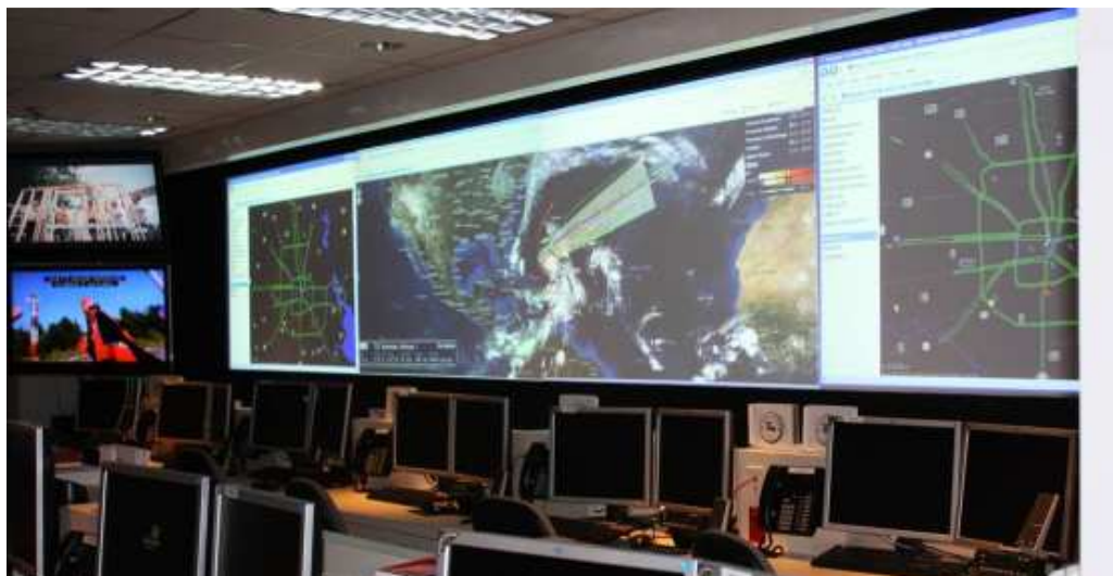
Figure 13: Emergency room TranStar
