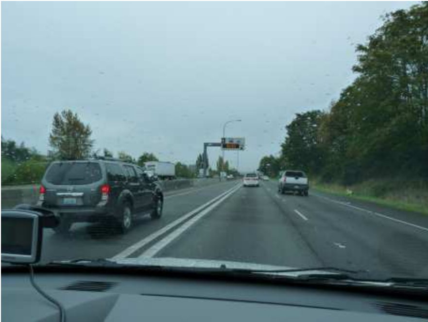
Figure 18: HOT Lane in Seattle
