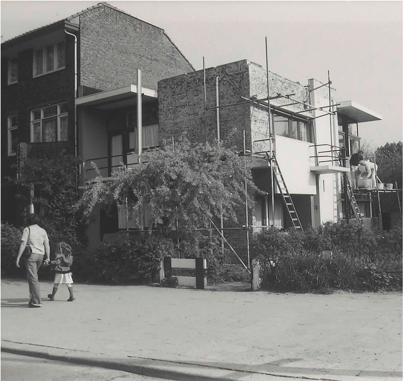
FIG. 1.12 South elevation (Prins Hendriklaan) with bare brickwork
