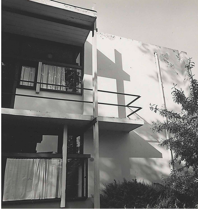
FIG. 1.2 Damage to the house became increasingly visible
