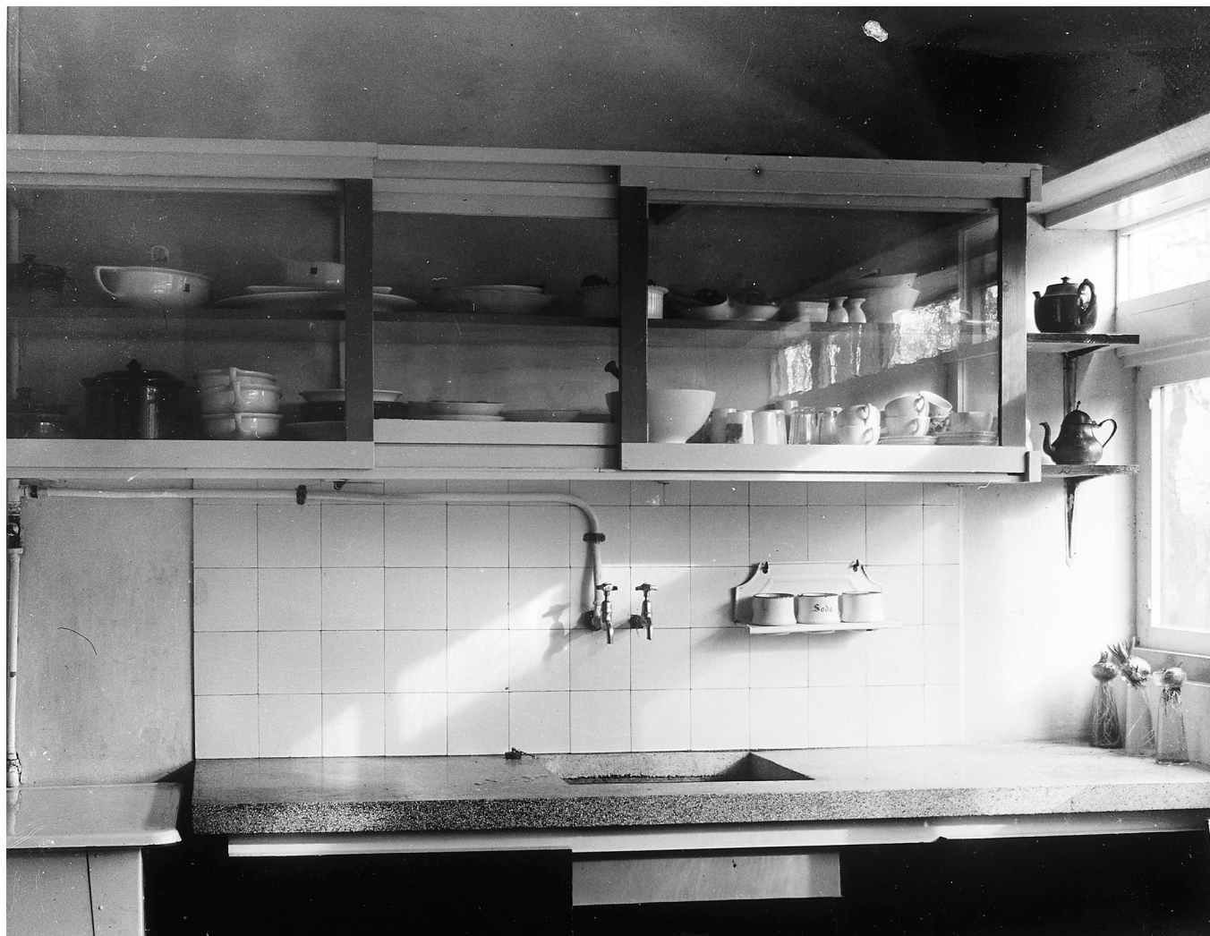
FIG. 4.44 Ground floor, kitchen, c. 1925
