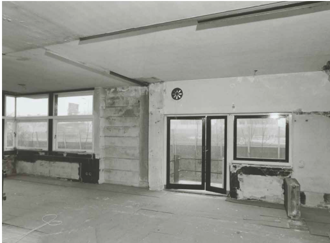
FIG. 3.3 The partially dismantled upper floor
