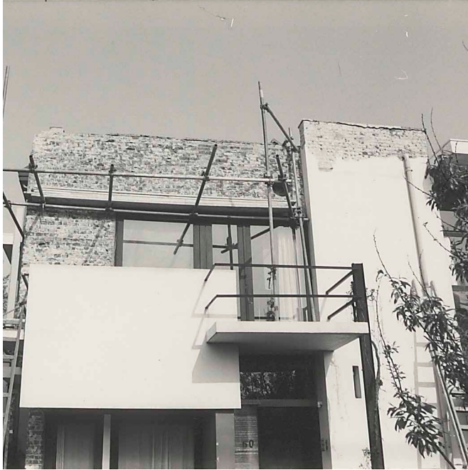
FIG. 1.13 East elevation with the plaster chipped away yet again
