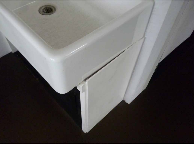
FIG. 5.2 Deformation of thin timber elements of furniture
