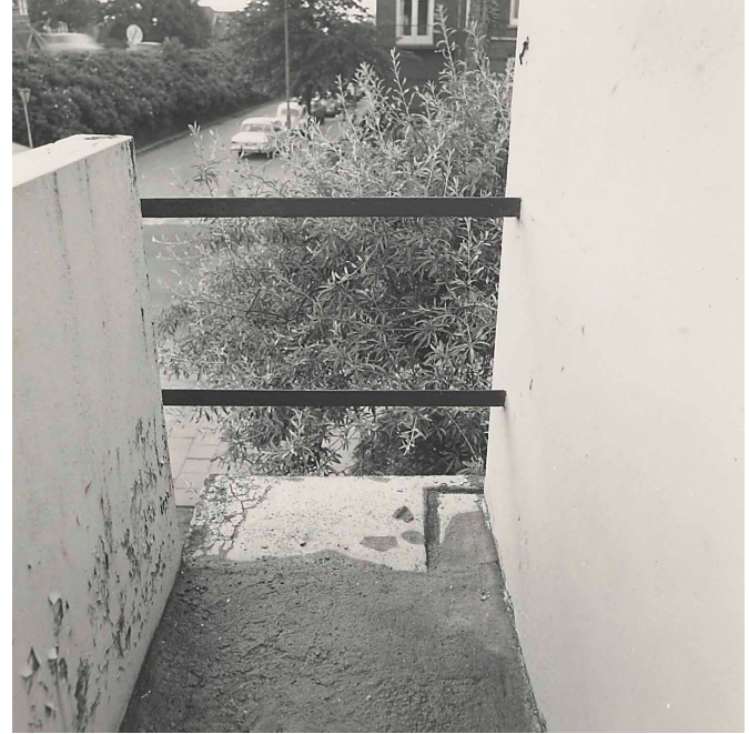
FIG. 1.5 After 50 years the concrete of the balconies also showed signs of cracks and damage
