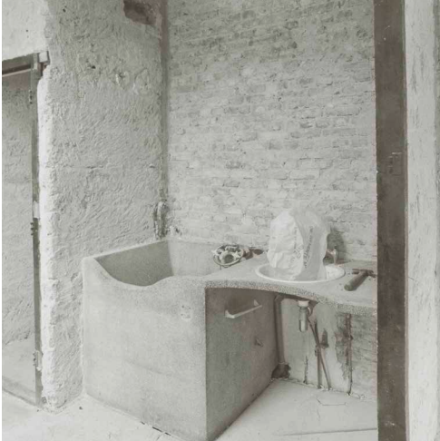
FIG. 3.7 Stripped bathroom with 'lavette'
