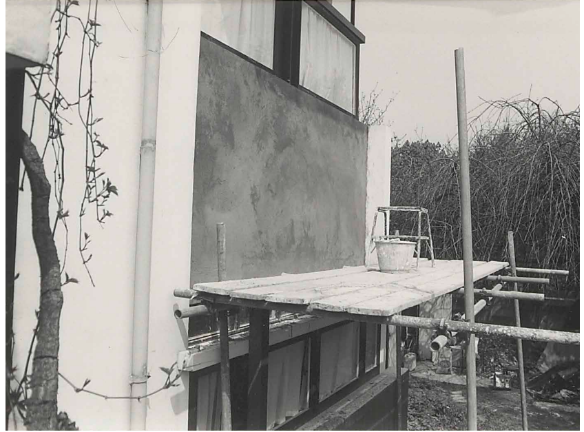
FIG. 1.11 After the plaster with hairline cracks was removed, the new render was applied in a single homogeneous coat
