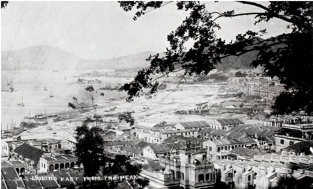
Figure 2.6 Completion of Wanchai reclamation by 1929
