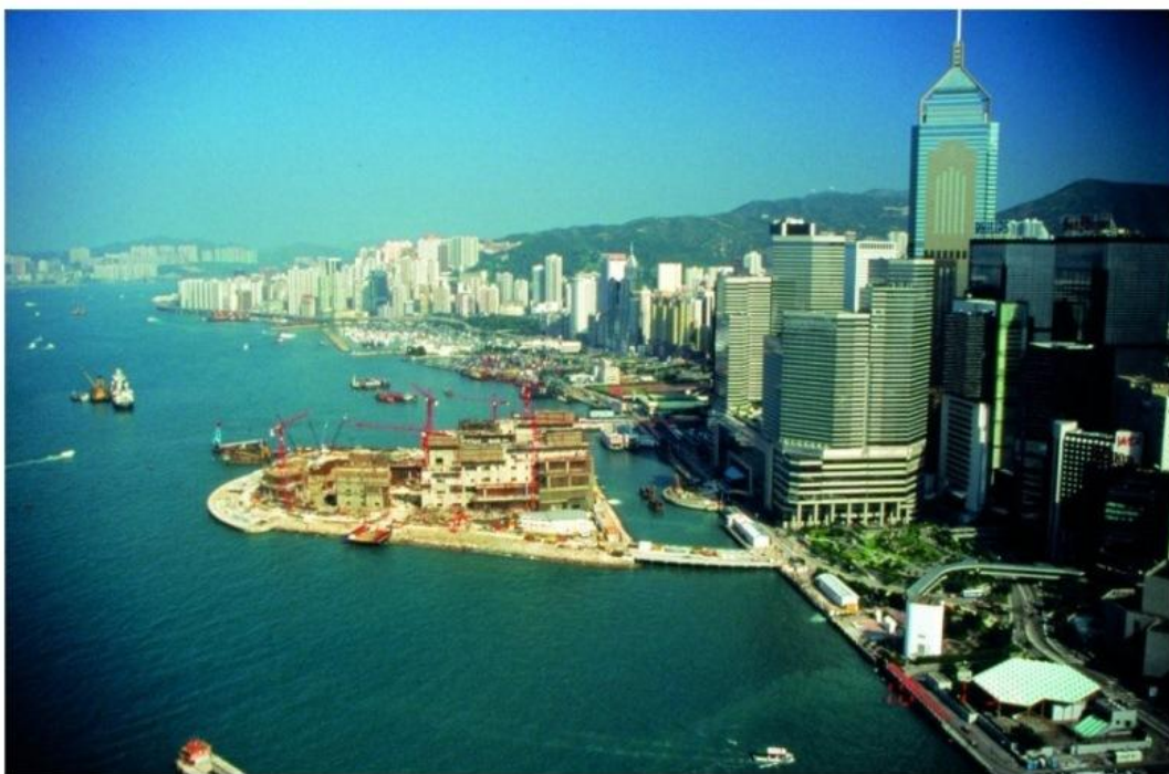
Figure 2.10 HKCEC Extension under construction, 1994
