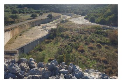
Figure 123: Channelized water imput of the Aposelemis dam 2023, photograph by author
