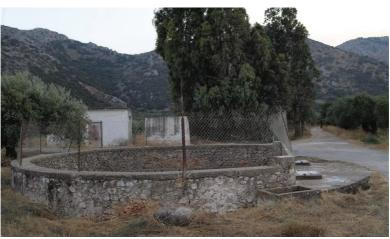
Figure 63: Public cistern used for water supply of the village of Lakonia in the eastern Crete, 1900. Source: https://www.slideshare.net/pergeo/brief-bistory-of-minoan-technologies-a-angelakis
