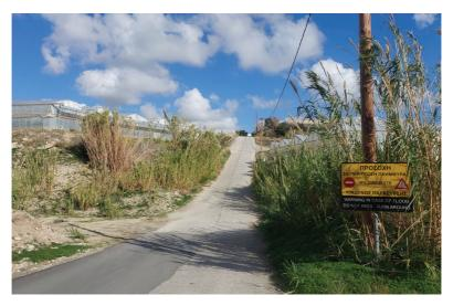
Figure 101: Road that crosses a river at Ierapetra (known as an Irish bridge), stays dry when the flow is low, but is designed to get submerged under high-flow conditions such as floods, photograph by author
