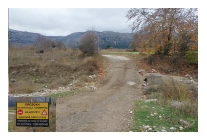
Figure 148: Road that crosses a river at Lasithi (known as an Irish bridge), stays dry when the flow is low, but is designed to get submerged under high-flow conditions such as floods, photograph by author
