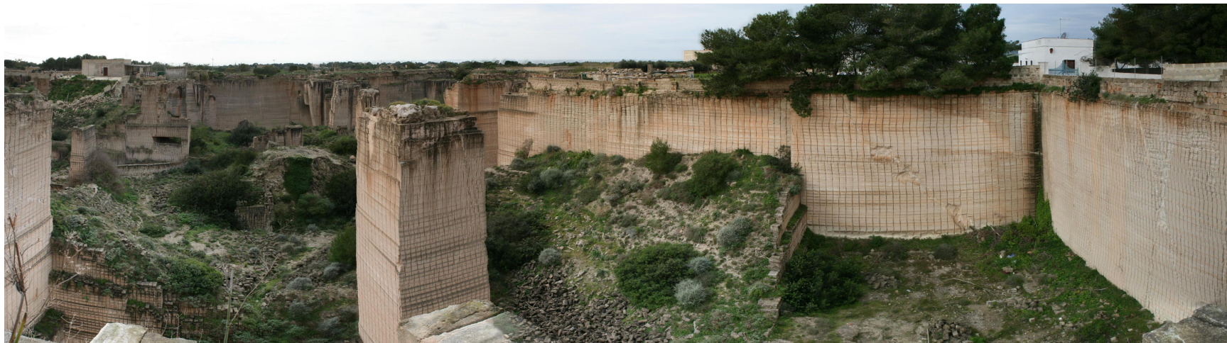
Figure B.6 – Abandoned quarry south of the Scalo Cavallo cliff to illustrate the general thickness of the calcarenite. Note the 'skyscraper' left behind in the centre of the quarry, which is about 20m high.
