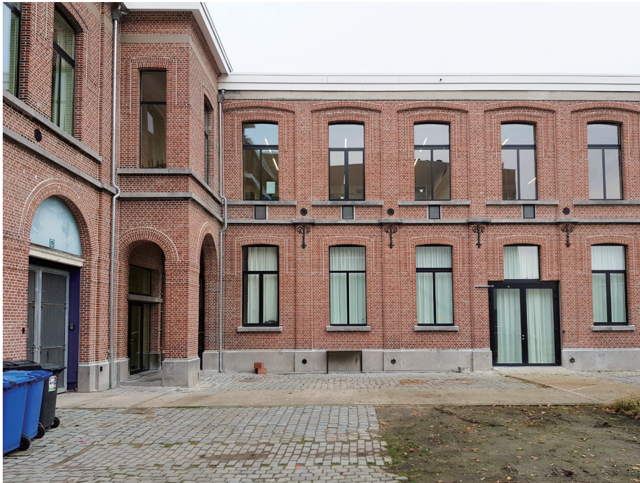
Internal facade of Academie Berchem
