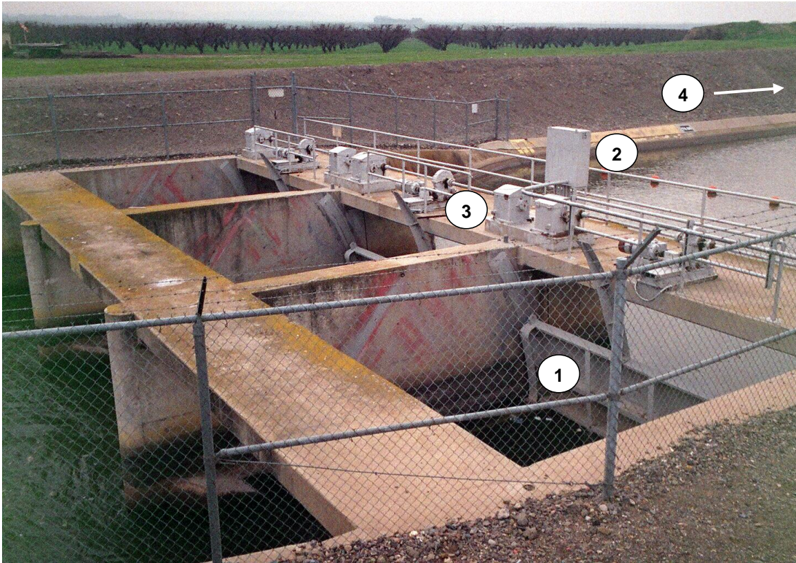
Figure 1.3 – Automated radial gate; 1: gate, 2: controller, 3: actuator, 4: pressure transducer Location: Delta Mendota Canal, Check structure 14, January 2004
