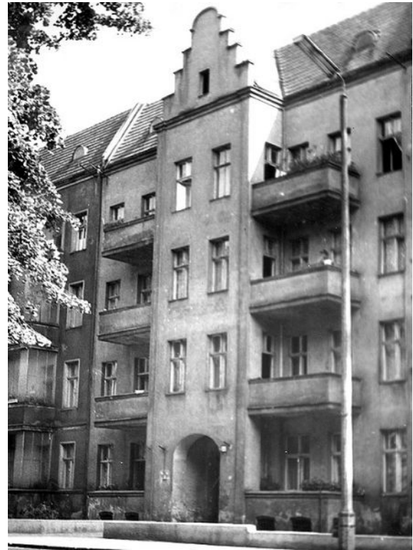
FIGURE 18. Unknown. (1950). [Photograph of National Unity tenement house no. 34 reconstruction after World War II]. Sedina.pl. Retrieved from http://sedina.pl/galeria/displayimage.php?album=1418&pid=13616#top_display_media
