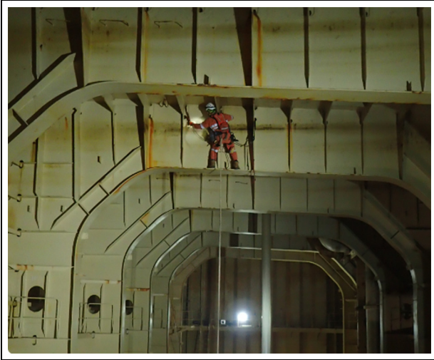
Figure 1. Hull inspection inside of Floating production and storage unit (FPSO) tank. 4
