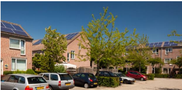
Fig. 12. Some of the smaller measures for an improved energy performance are visible in parts of the Stedenwijk midden by Ymere. Especially all PC-cells.
