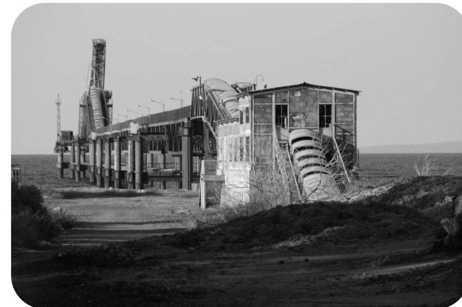
RAILWAY FROM MINES TO HARBOURS
